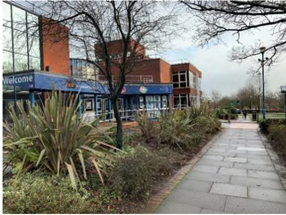
Photo 1 – Campus west north main building and entrance.
