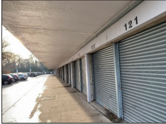
Photo 13 – Garages assessed for bat roosting potential.
