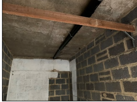
Photo 14 – Interior of garages.
