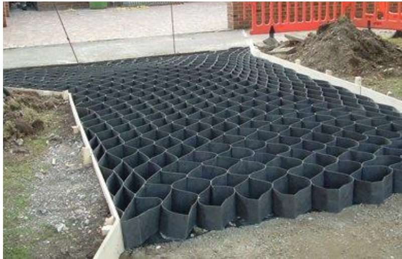
Image 10 - Cellular no-dig system: Photo shows above ground cellular load spreading system for installation of permeable hard surfaces close to trees. In this case the cellular system is shown before being filled with clean angular stone. Note the permeable geotextile preventing the stone migrating to the ground beneath
