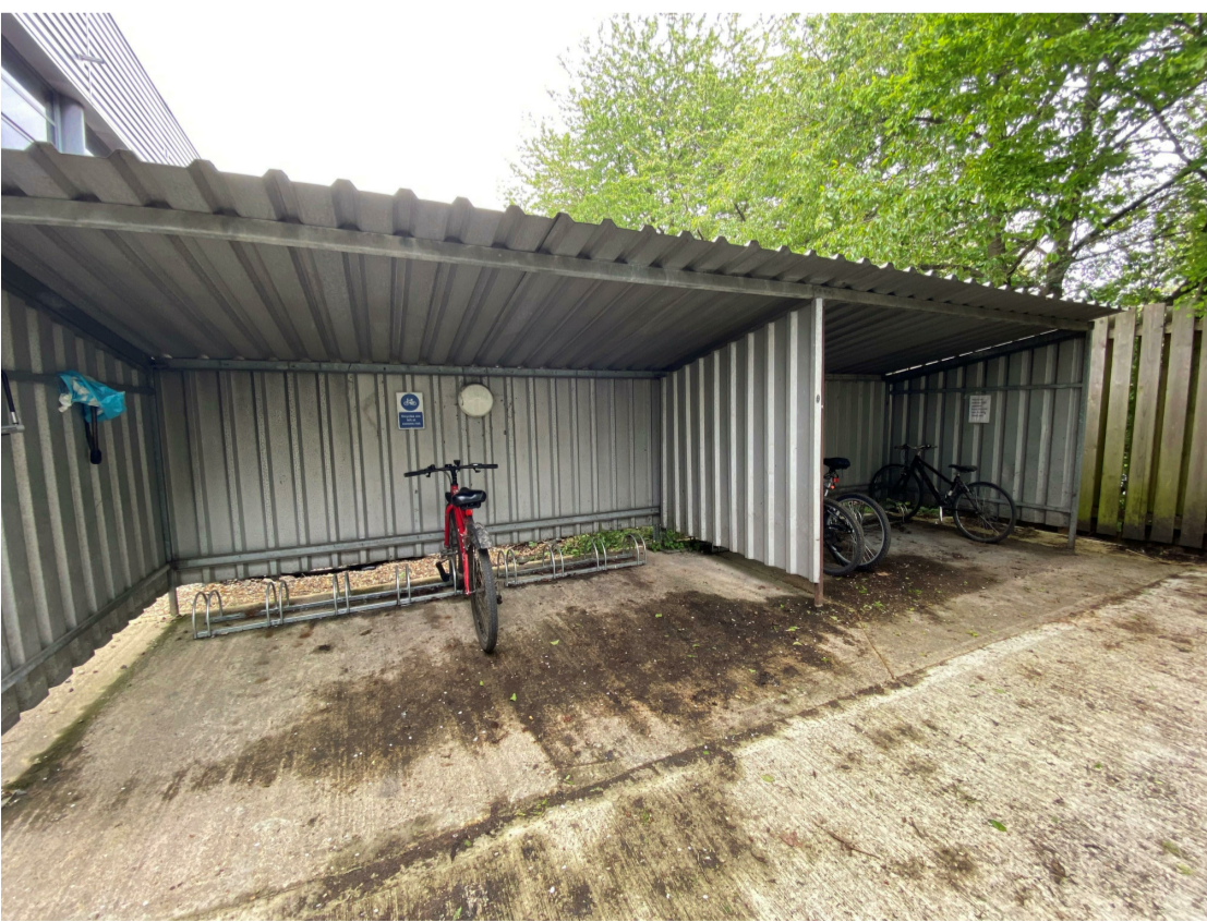
4 Aquarius house existing bike rack
