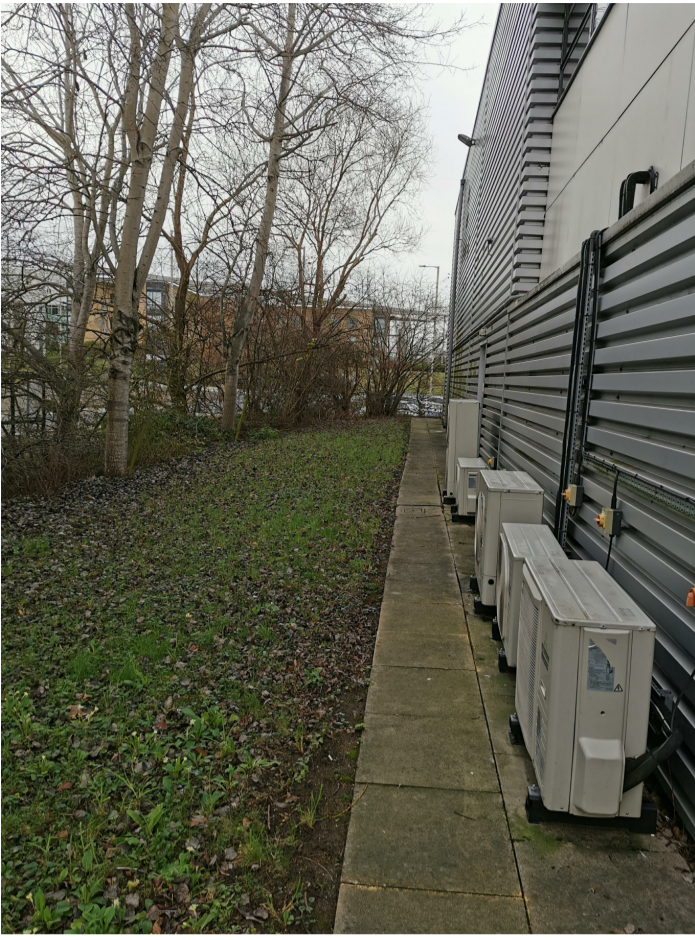
1 View from front of the building
