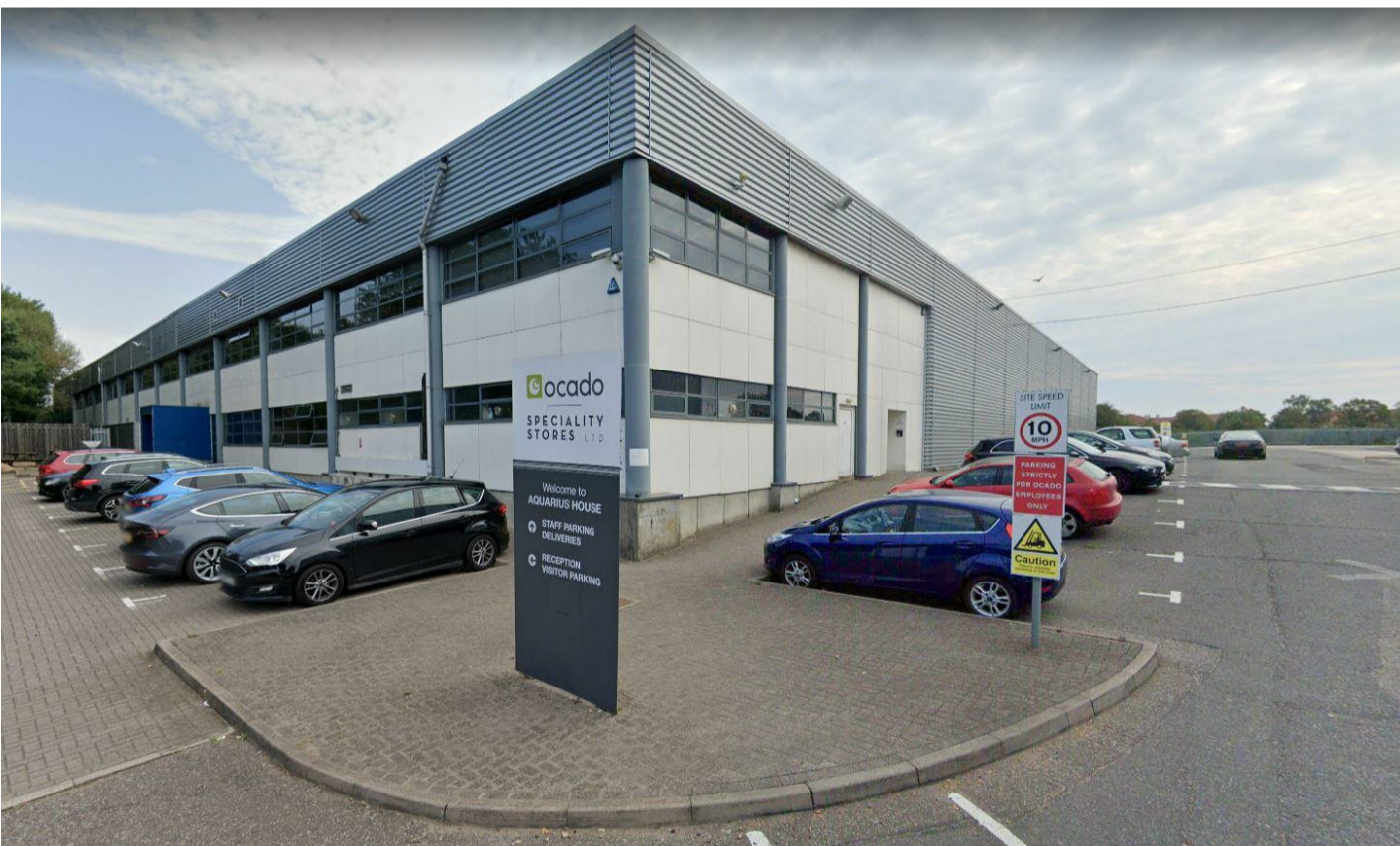
3 View of Aquarius house from the site entrance
