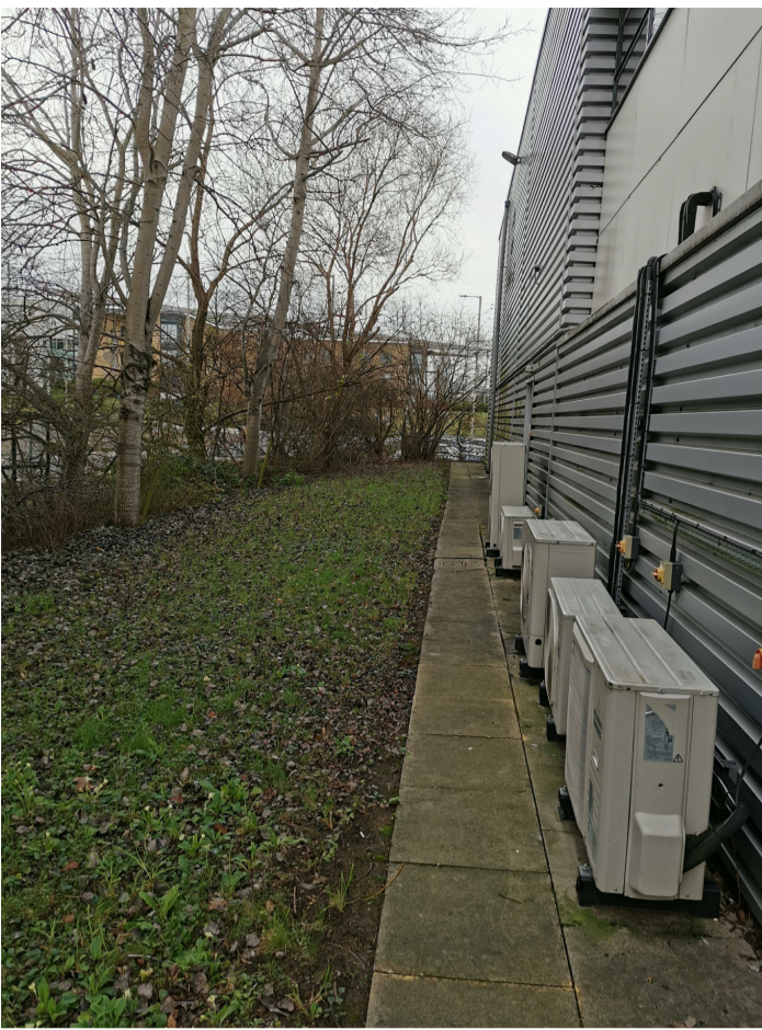
1 View from front of the building
