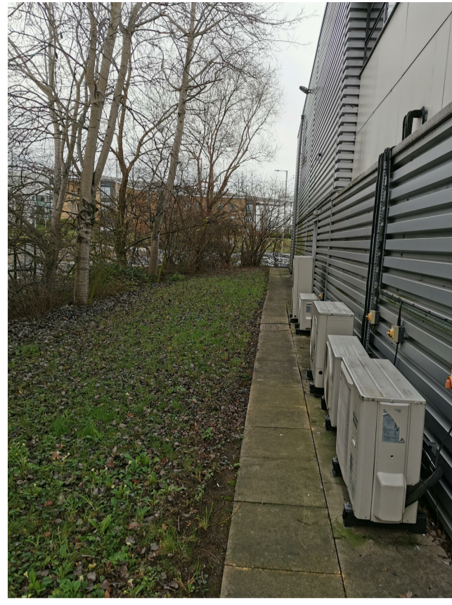
1 View from front of the building
