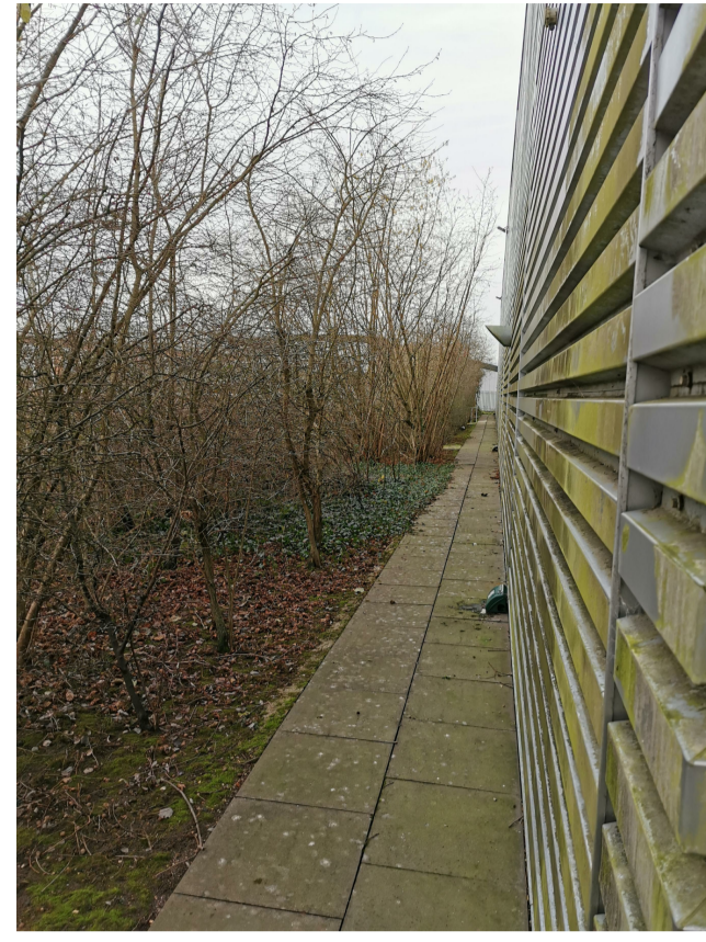
2 View from side of the building where new fire escape is being installed
