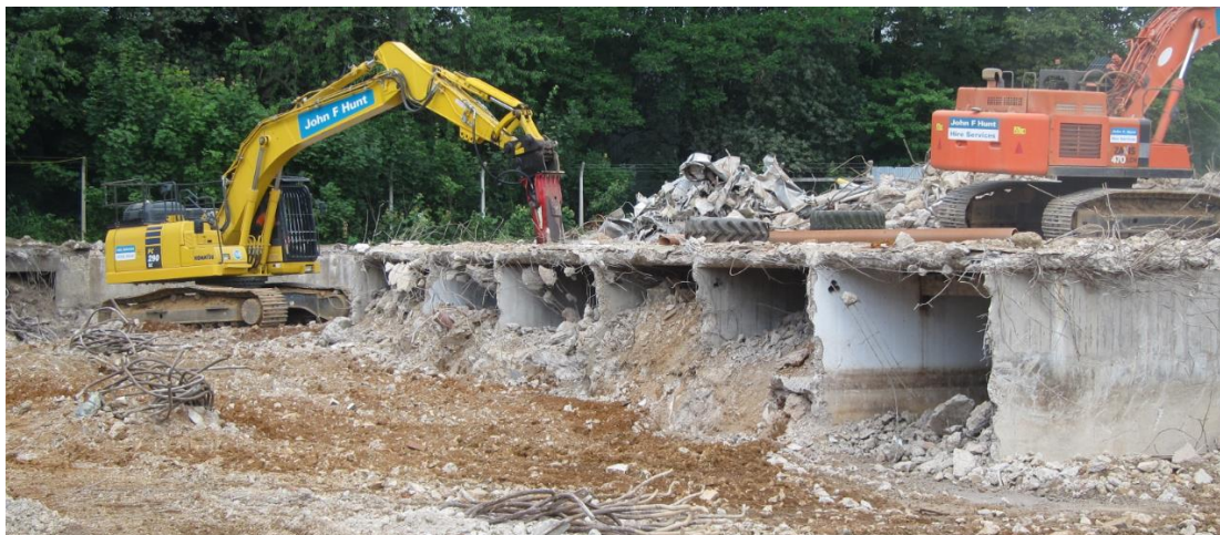
Photograph 2-4: Demolition of the firing range tunnels
