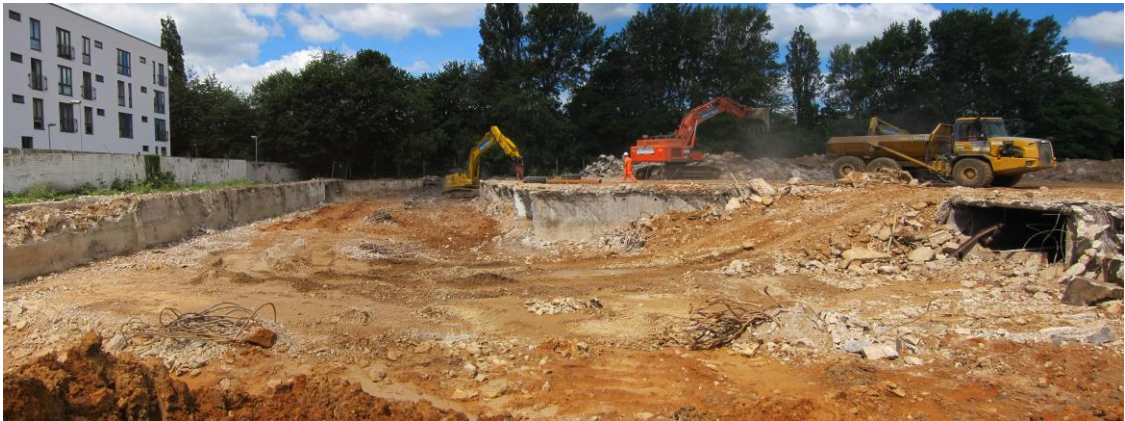
Photograph 2-5: Demolition of the firing range tunnels and basement
