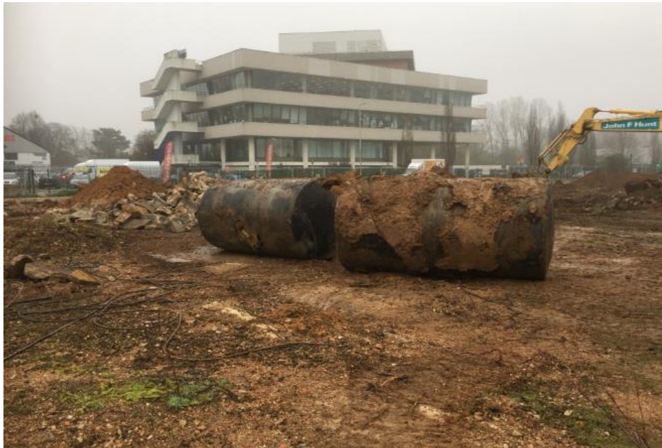
Photograph 2-2: USTs removed from southern site
