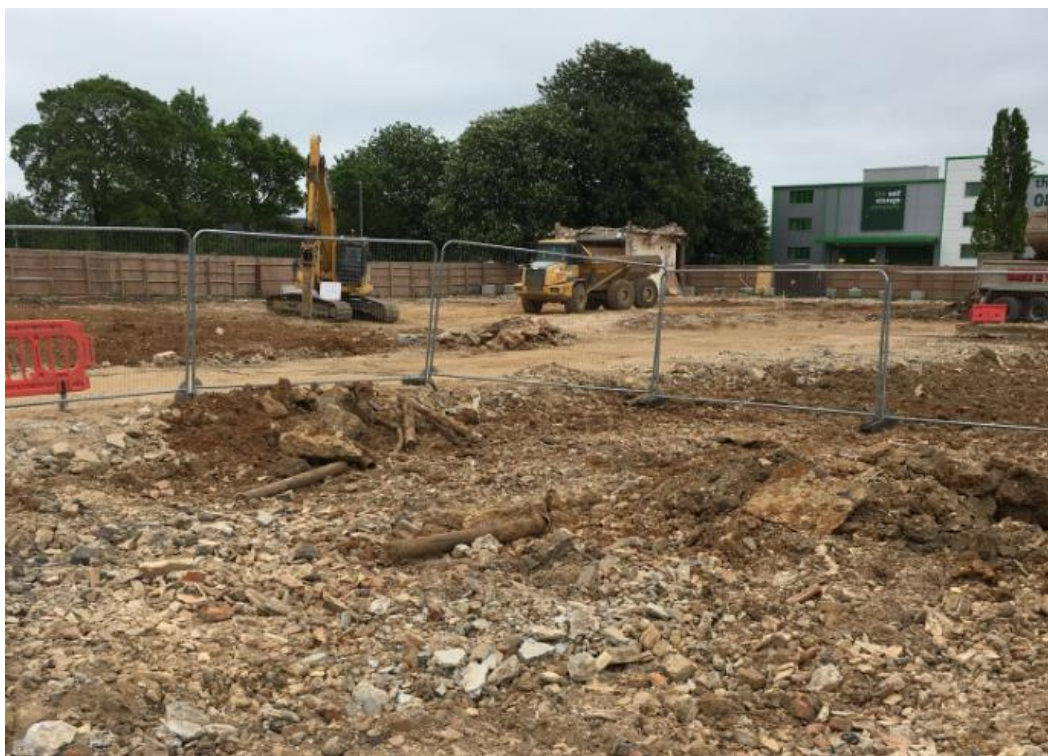
Photograph 2-7: Quarantine area with visible cement-based ACMs
