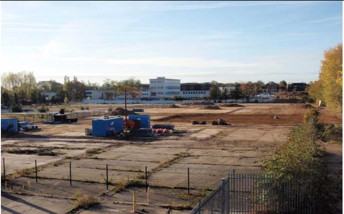
Former Polycell factory area following removal of groundwater treatment system and backfilling of the tank farm excavation.
