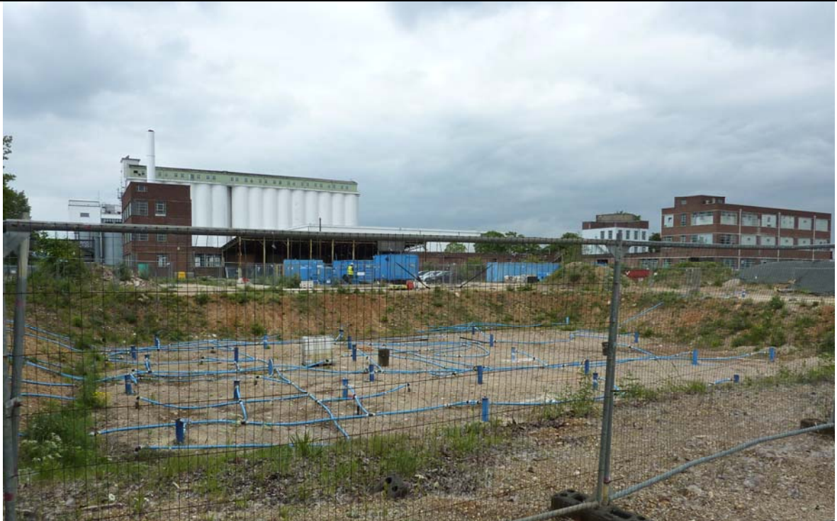
Polycell factory tank farm area – groundwater treatment system in operation following removal of tanks and impacted soils.
