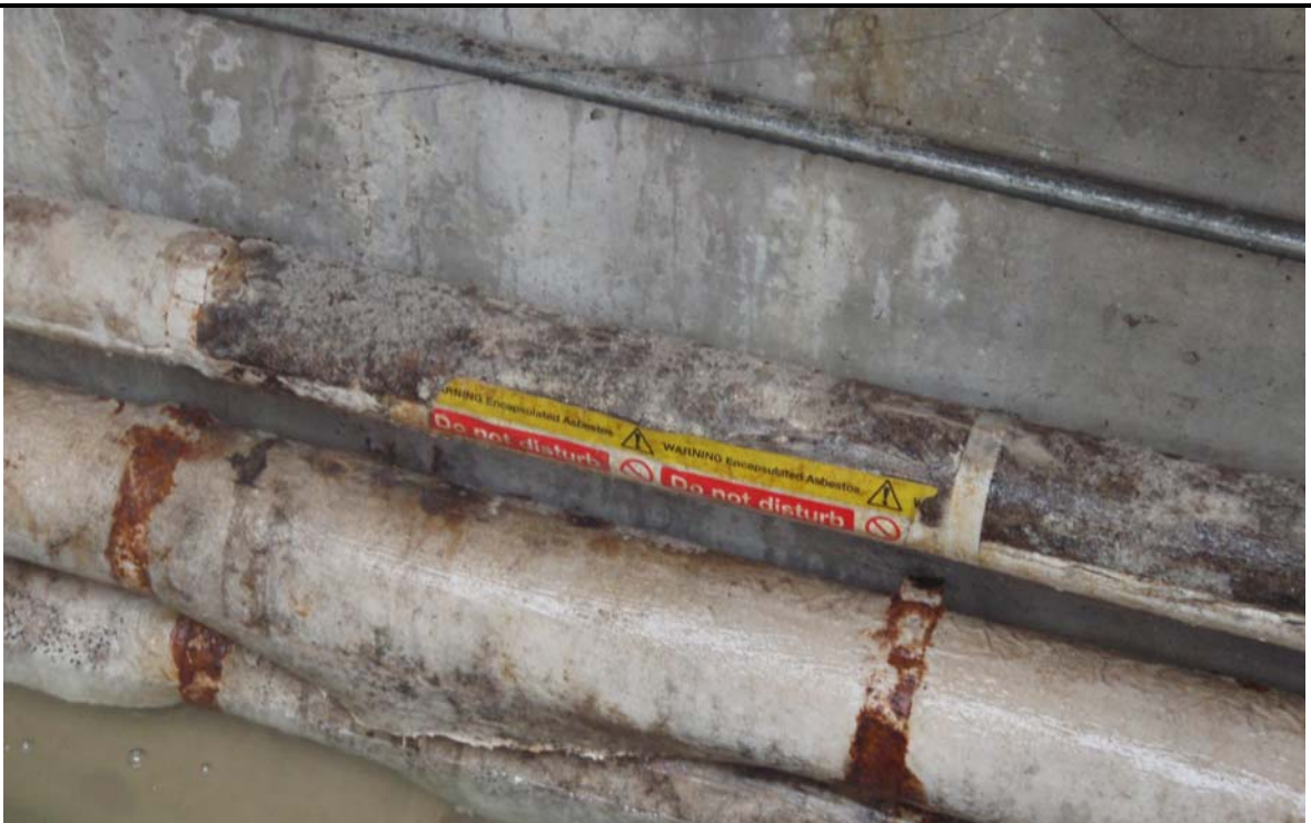
Lagged pipe and asbestos warning signage in water filled service duct in the south of the Site.
