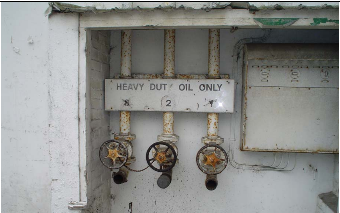
Fuel oil tank fill points associated with the Polycell factory boiler house.
