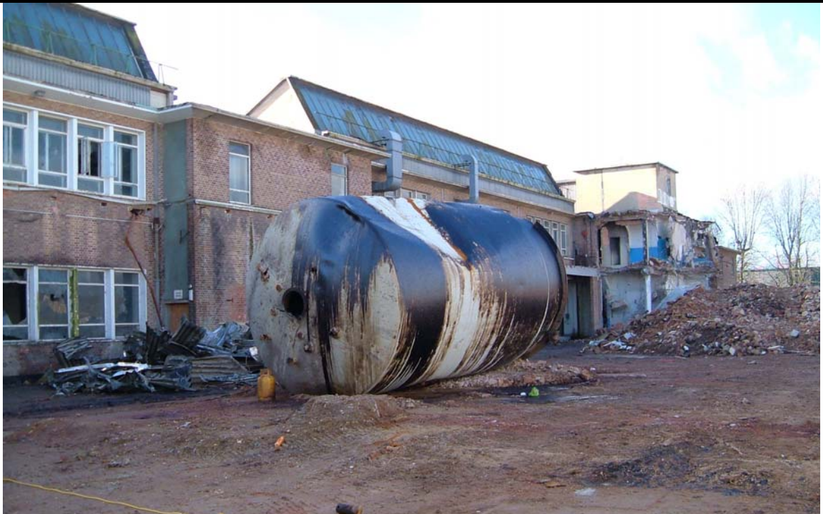
Fuel oil tank associated with the Polycell factory boiler house during demolition.
