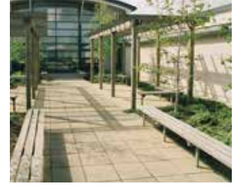
Area: Podium & Roof gardens Type: Concrete flags Size: 600x600mm Colour: Buff / light grey
