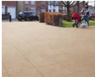
Area: Private amenity Type: Concrete Flags Size: 400x400mm Colour: Natural
