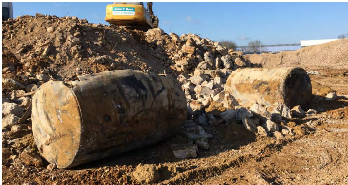
Photograph 2-5: USTs removed from rear of silos
