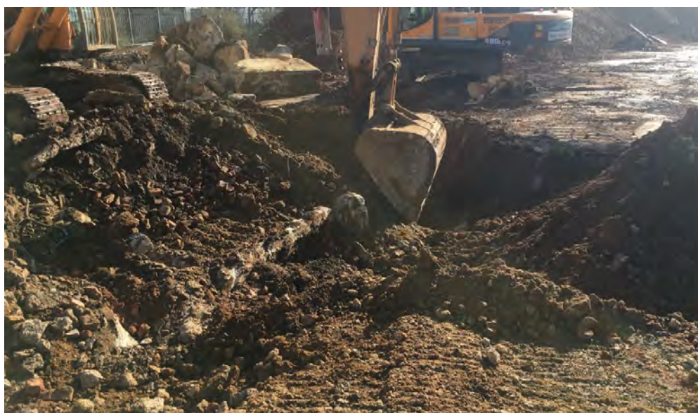
Photograph 2-8: Slab removal in area of possible historic ASTs
