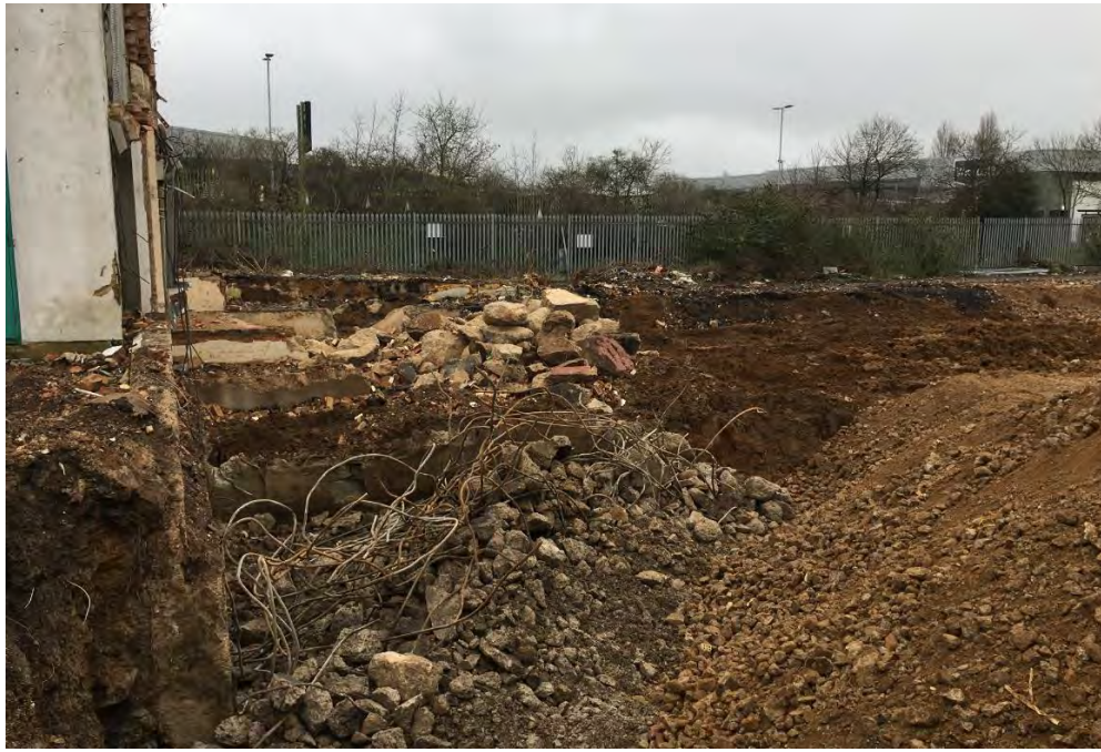
Photograph 2-9: Slab removal adjacent to 11kV substation
