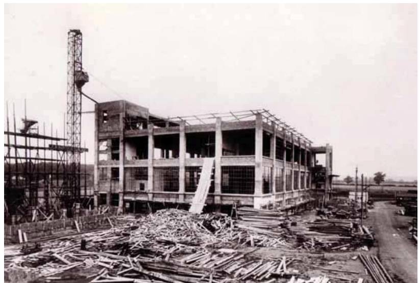
Figure 9: Showing the construction of the reinforced concrete Shredded Wheat Factory c.1924 [© Welwyn Garden City Heritage Trust website]
