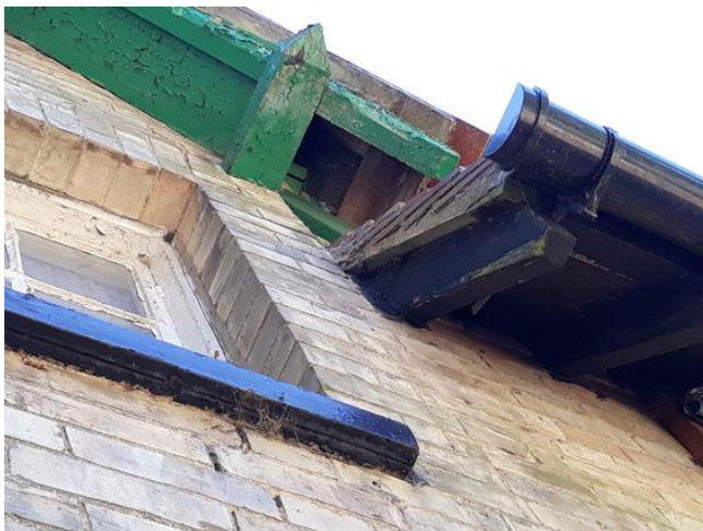
Photograph 6 – Access into eaves of main building
