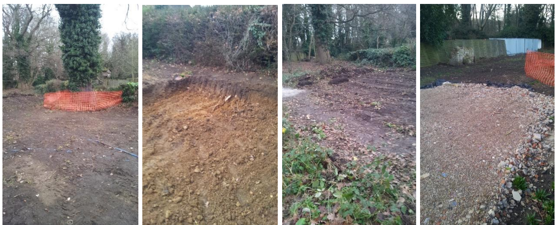
Photos - showing the construction of 52 Bridge Road Driveway adjacent to TPO Oak Tree. This drive was subsequently re-laid in accordance with the approved plans & more recently dug out again within the root protection area-
