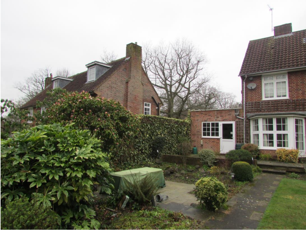
Rear view of no. 39 Sherrardspark Road showing dormer windows added to rear roof slope
