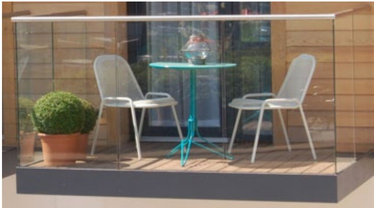
9. Balconies: Balcony Life Ltd, Vista View frameless glazed balconies with 10mm toughened glass- clear and obscured glazed where appropriate- See proposed elevations.
