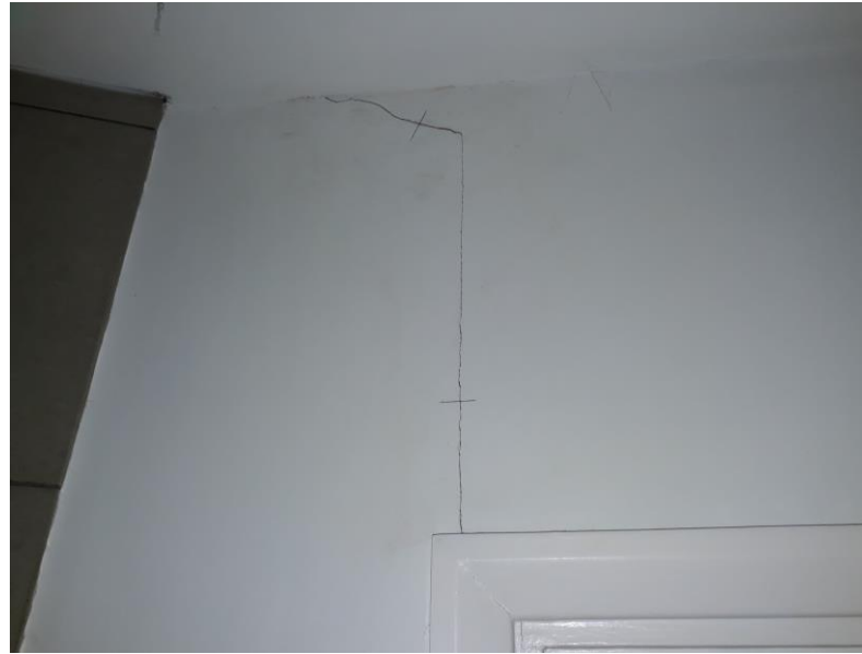
Max 1 mm wide crack - above bathroom door first floor rear
