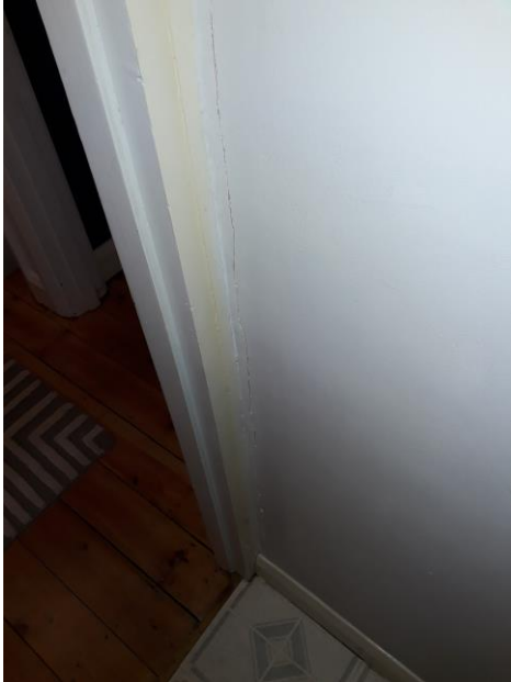
Vertical 1 mm crack on kitchen side adjacent to hall
