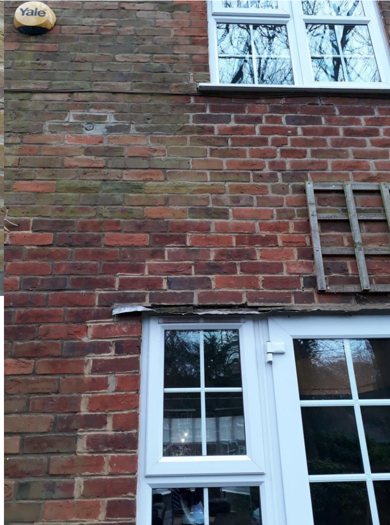
Minor stepped cracks rear elevation - evidence of previous works pre dates Insured's occupation
