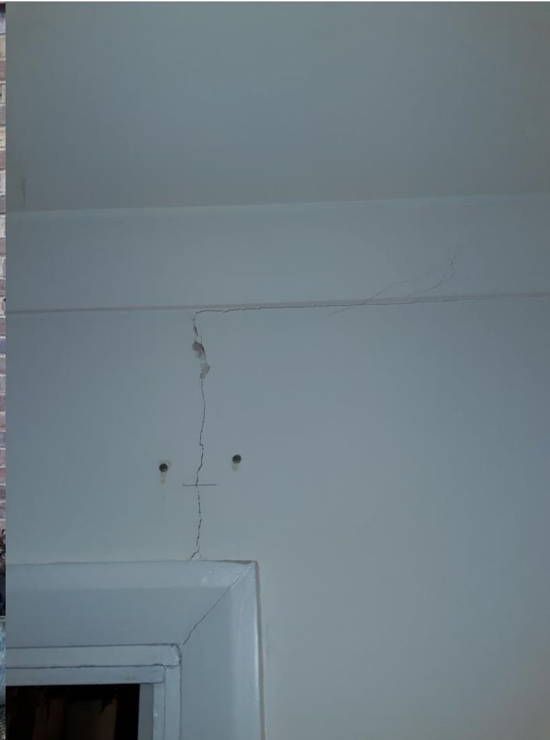
1 mm wide crack above door from hall into kitchen beyond
