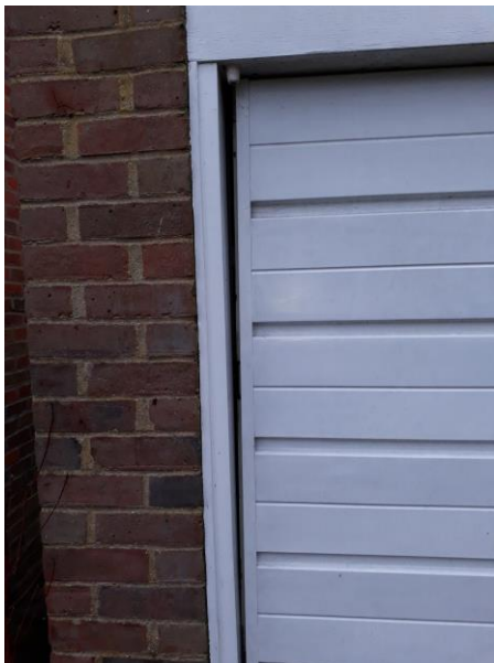
Close up of gap to garage up and over door
