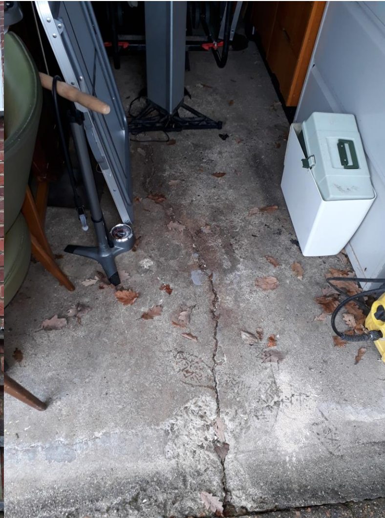
Crack in garage floor
