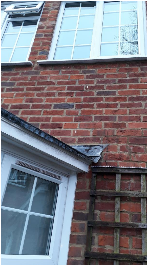
Minor stepped cracks on front elevation below first floor window
