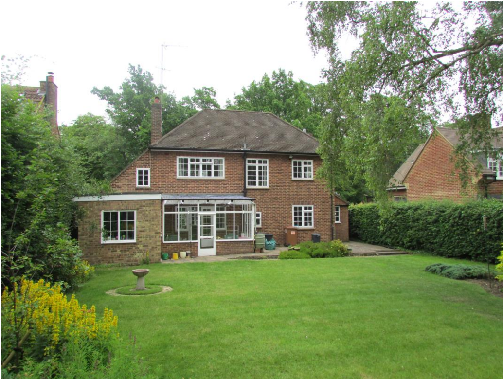
Rear view of house, showing modern conservatory to be demolished
