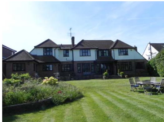
Photograph 6: Rear (north) elevation
