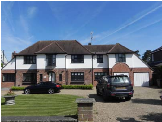
Photograph 5: Front (south) elevation
