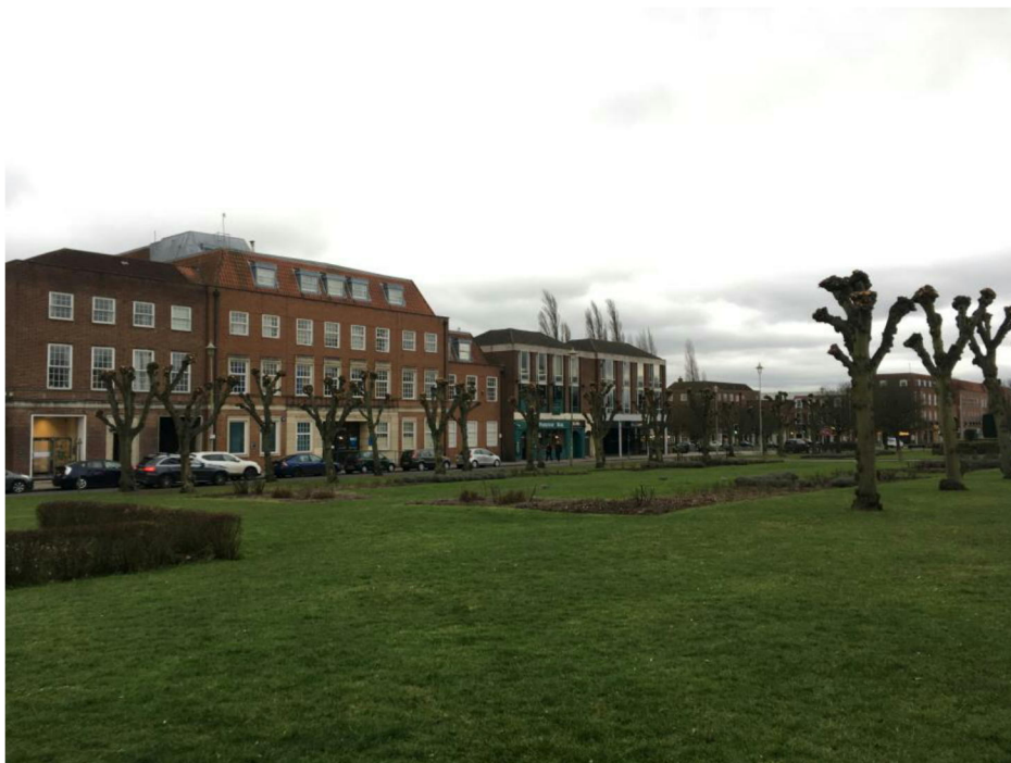
Photograph 6: Site viewed in context of Parkway
