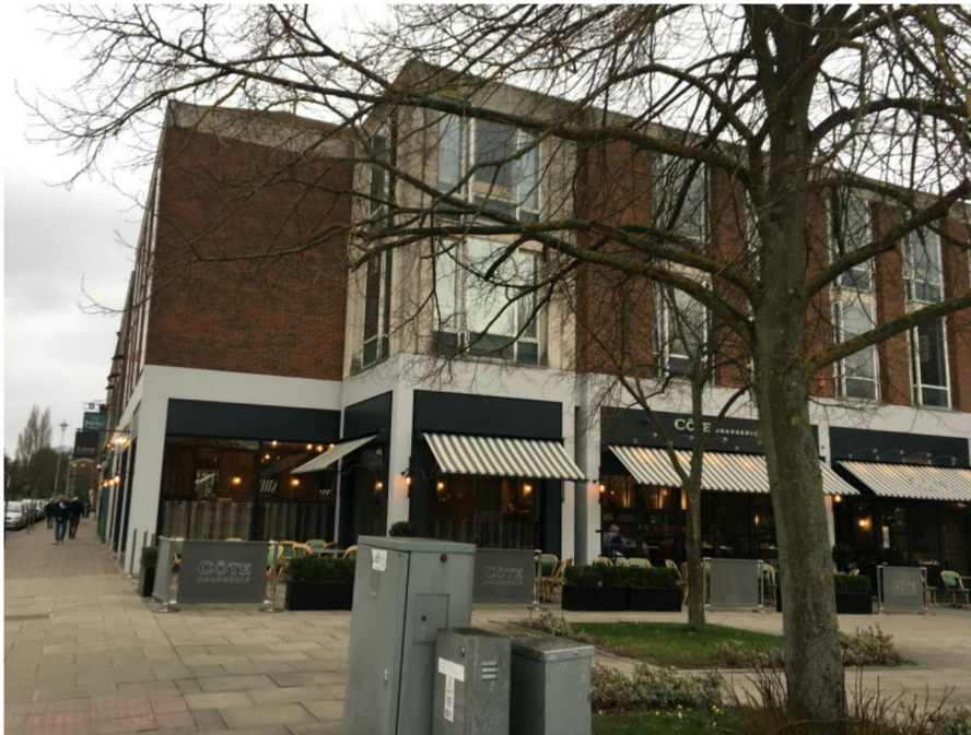
Photograph 3: Corner of building inset at junction of Howardsgate and Parkway
