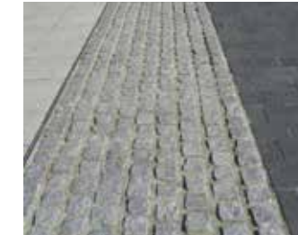
Area: Road entrances Type: Granite setts Size: 100x100x100mm Colour: Silver grey
