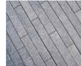
Area: Goodman Square Type: Granite linear planks Size: 200mm width x Random lengths Colour: Mixed greys
