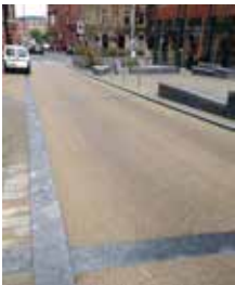
Area: The Weave Type: Asphalt surface dressed with gravel chips in resin Colour: Buff
