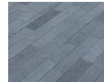
Area: Reiss Walk Type: Concrete blocks Size: 300x100mm, 200x100mm Colour: Mixed greys
