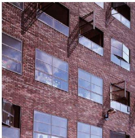
Kollhoff Architekten. Piraeus apartment building. Amsterdam, Netherlands. Completed 1994. Planar façade with steel-framed windows.
