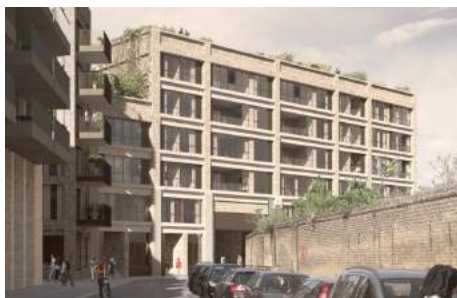
Hawkins Brown. White Post Lane. London. Ongoing. Structural frame expressed and infilled with curtain wall panels with horizontal emphasis.
