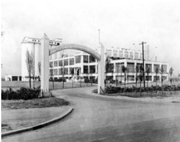
Figure 20: The Folly Arch – the entrance to the ‘Home of Shredded Wheat’
