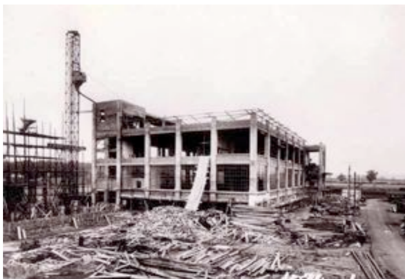
Figure 9: Showing the construction of the reinforced concrete Shredded Wheat Factory c.1924 [© Welwyn Garden City Heritage Trust website]
