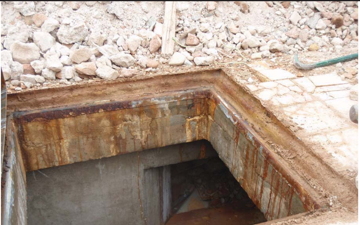
Voids/ducts in the south-west of the Site.
