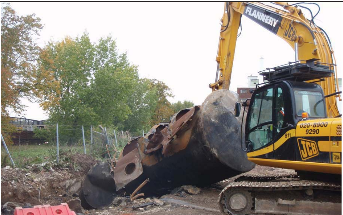
Polycell factory tank farm area during remediation works.
