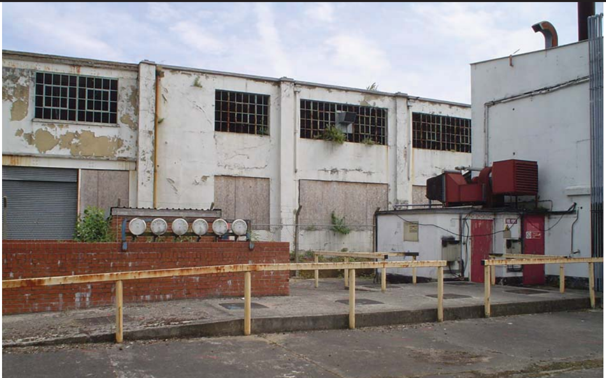
Polycell factory tank farm area prior to demolition.
