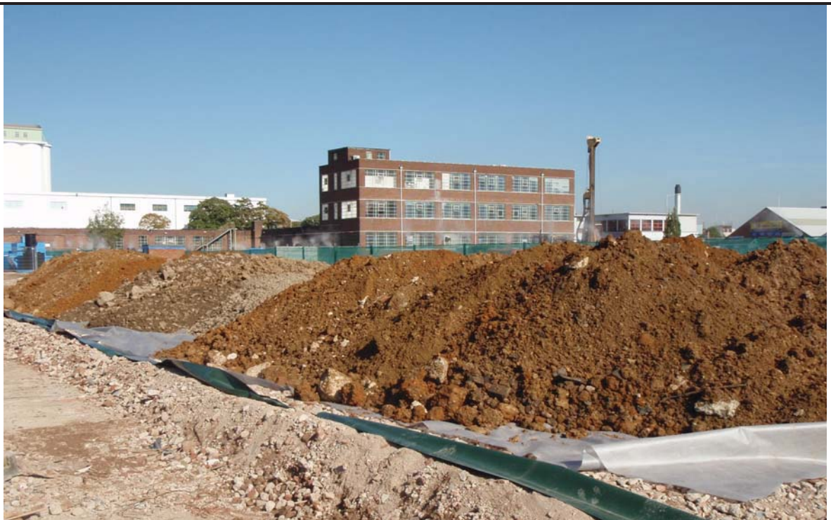
Excavated soils from the tank farm excavation on biopiles for treatment.
