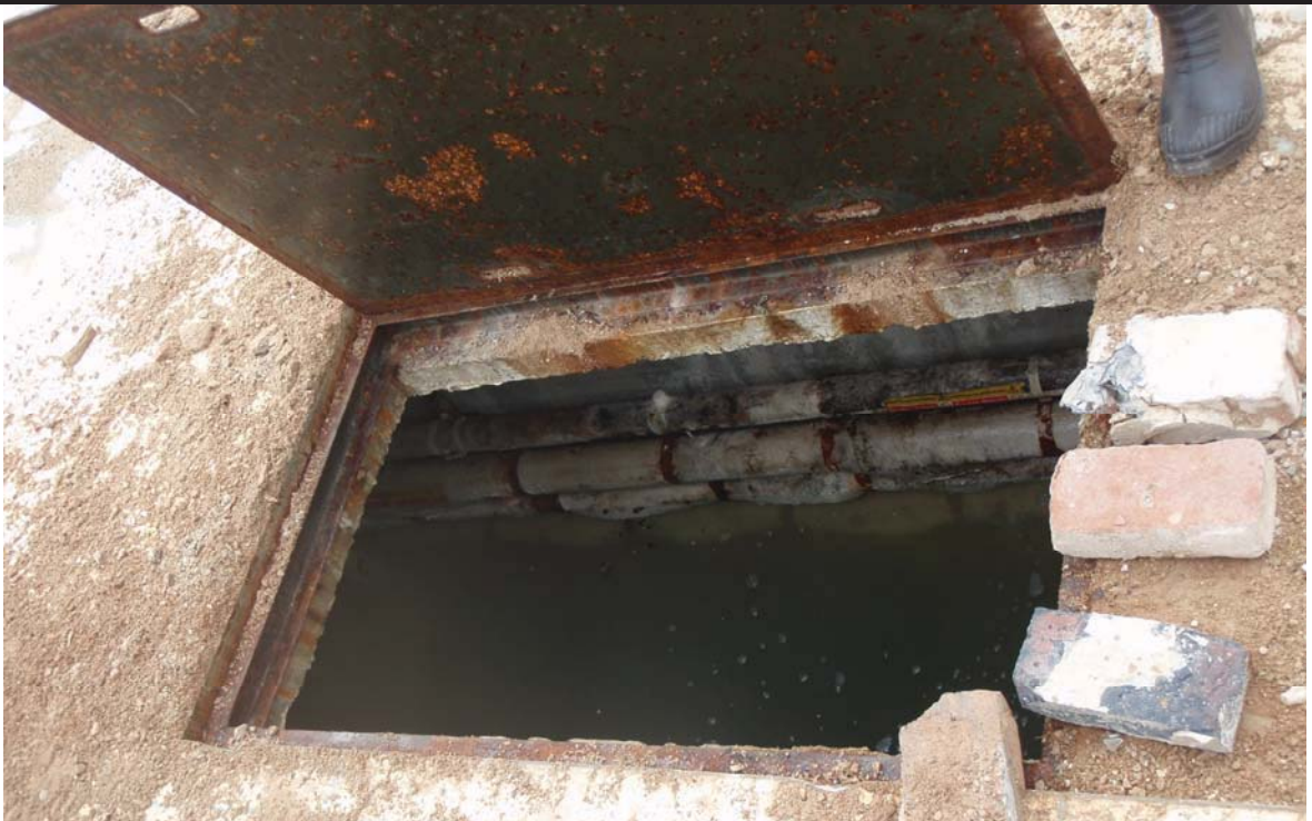
Water filled service duct in the south of the Site.
