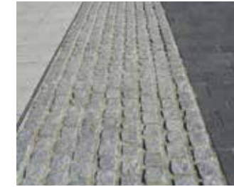
Area: Road entrances Type: Granite setts Size: 100x100x100mm Colour: Silver grey
