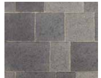
Area: Public realm & Residential block entrances Type: Concrete flags Size: 200x200mm, 200x300mm Colour: Mid grey
