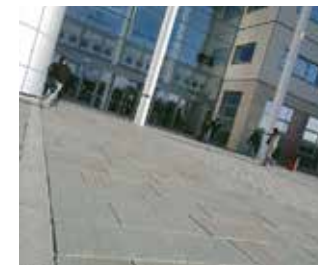
Area: Louis De Soissons Type: Concrete flags Size: 900x300mm Colour: Mid grey
