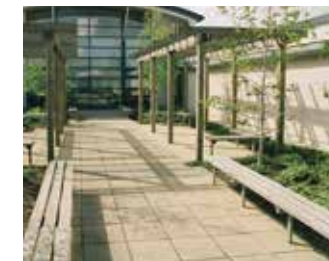
Area: Podium gardens Type: Concrete flags Size: 600x600mm Colour: Buff
