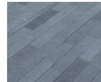
Area: Reiss Walk Type: Concrete blocks Size: 300x100mm, 200x100mm Colour: Mixed greys
