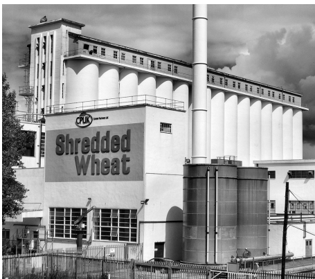
Signage facing the railway
