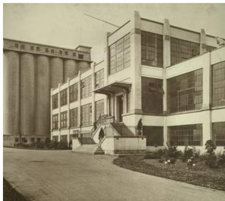
Production Hall – original east elevation
