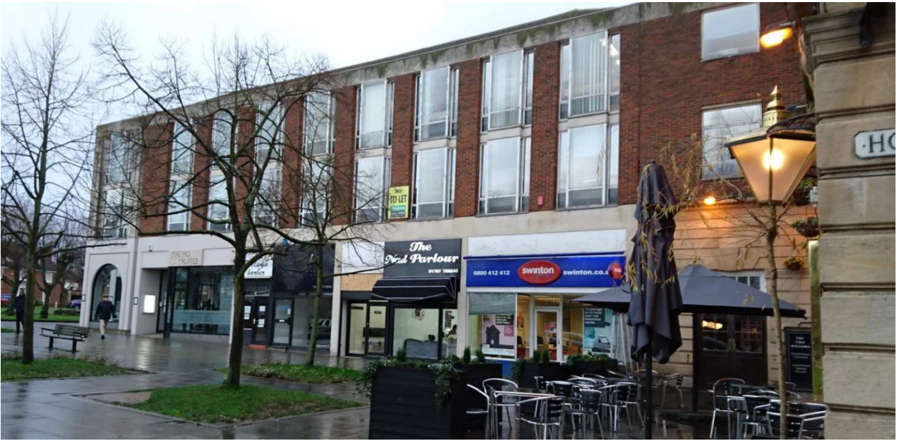
Picture 1: Existing steel windows on 1 st and 2 nd floor
