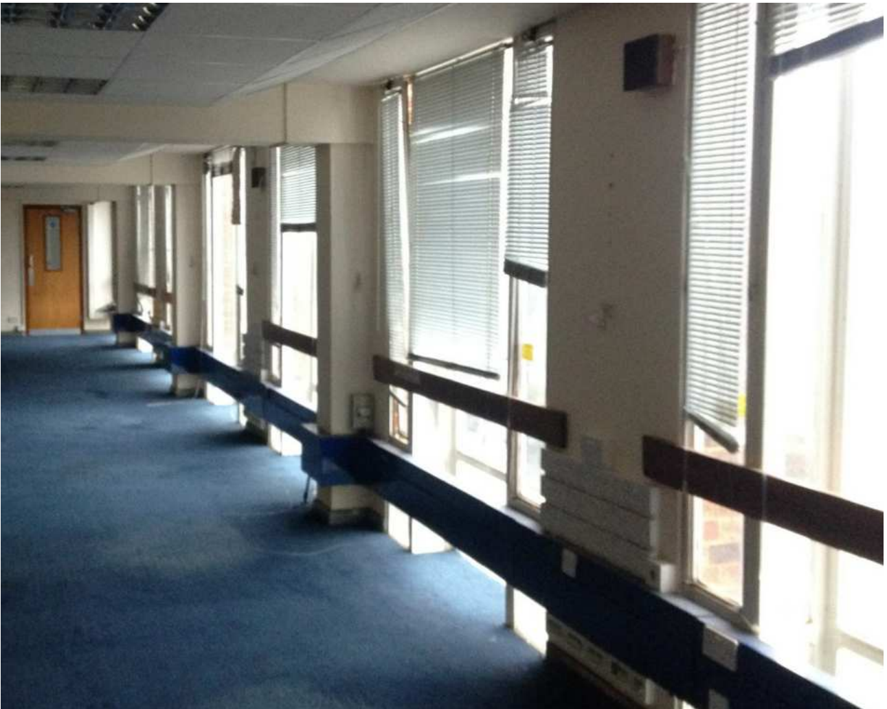
Picture 2: Existing windows from inside
