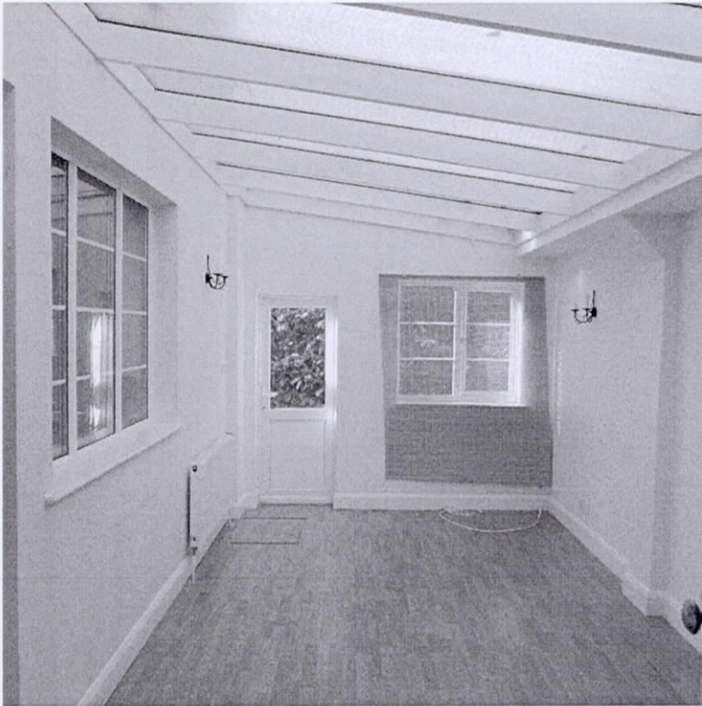
Sloping polycarbonate roof to existing breakfast room
