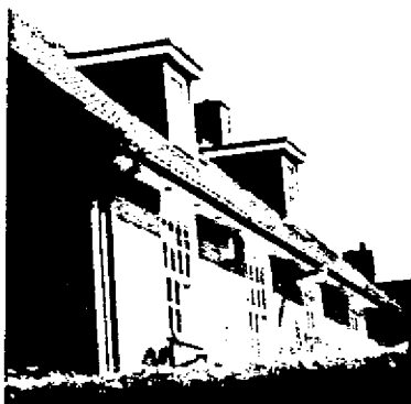
Dormer windows in adjacent properties
