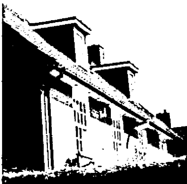
Dormer windows in adjacent properties
