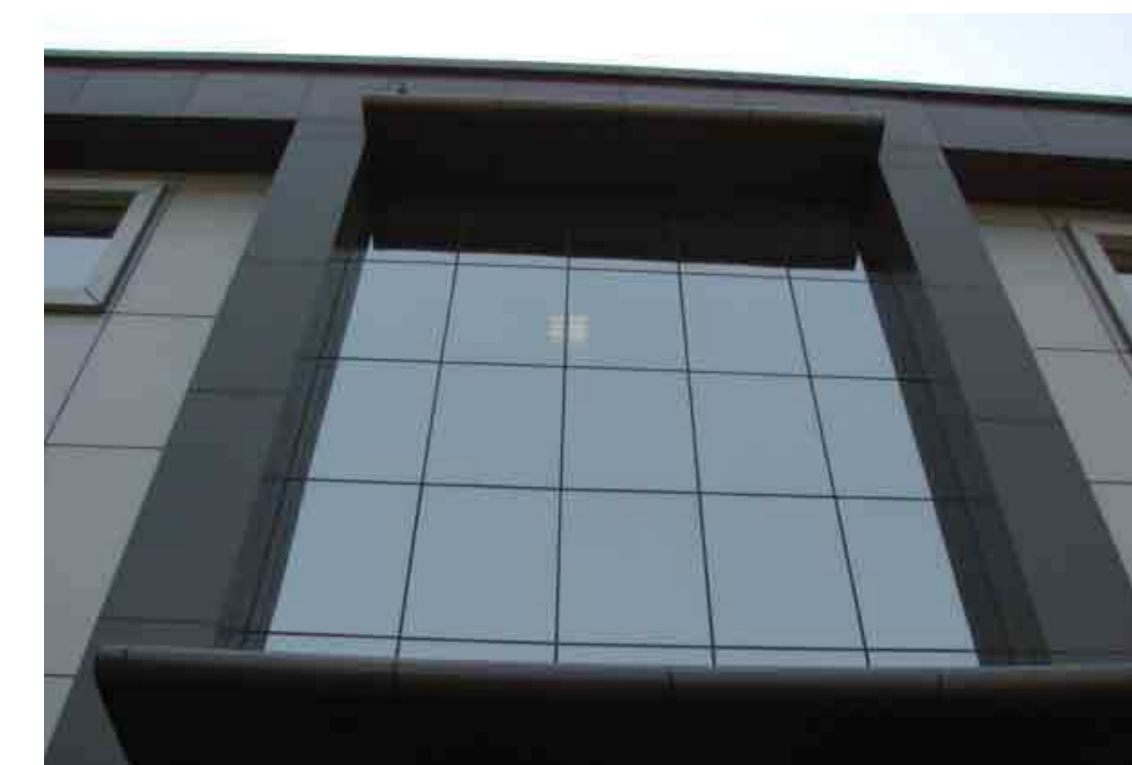
Feature glazing system - Kawneer PF System with silicon joints between panels. Glass tinted for solar control.
