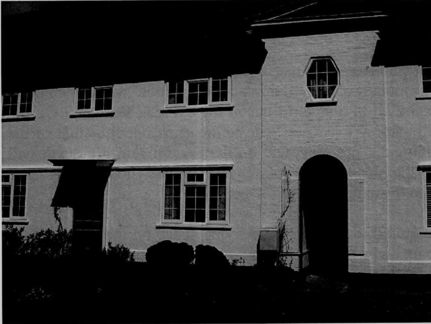
1) The existing front elevation.
