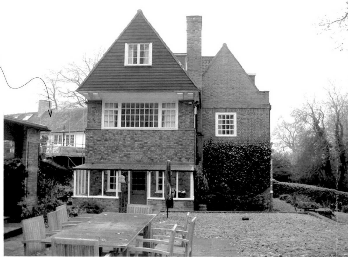
North Corner of Existing House Showing Adjacent Terrace & Edge of Poolhouse
