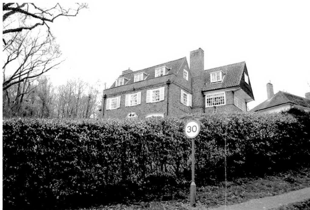
West Elevation of Existing House - View from Brockswood Lane
