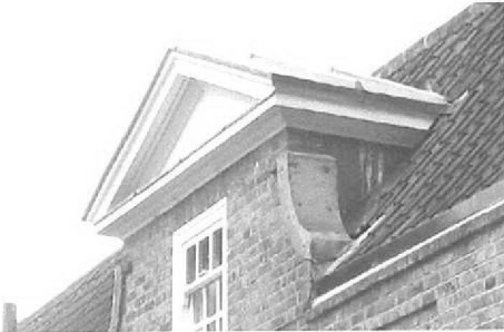
Example of existing lead roofing & flashings
