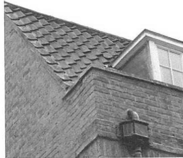
Example of existing parapet coping stone
