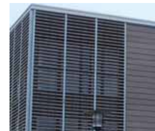
Metal solar shading
