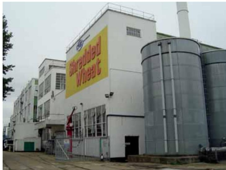
5 The boiler house burned coke to provide hot water and steam for cooking and cleaning processes that took place inside the factory.
