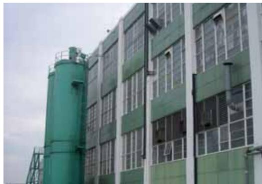
5 The external elevations do not differ very much from the traditional type of factory building having plain facades with the largest possible window openings set between vertical piers and horizontal transoms.
