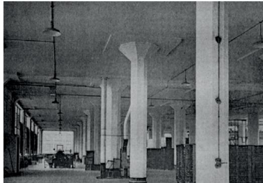
3 The advantage of basing the design of the factory on a mushroom system was the elimination of beams projecting below the ceiling and thus to enable maximum glazing of the external walls and an even distribution of natural light.
