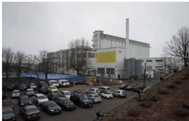
Figure 3.2: Former Shredded Wheat factory buildings - functional design, with informal composition of forms and large scale (production hall not visible)
