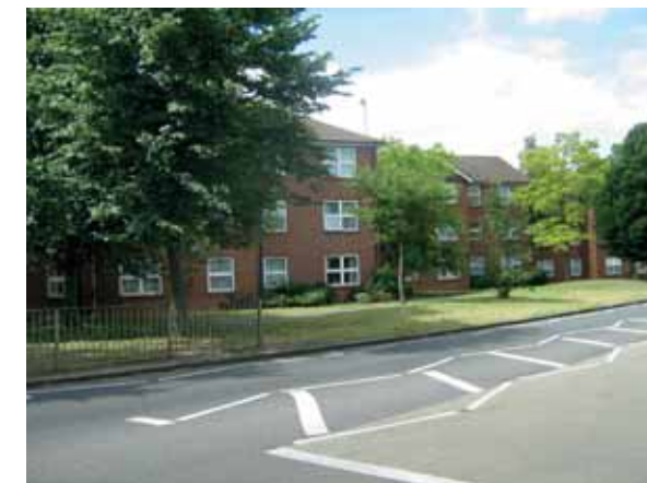
Existing housing on Broadwater Road within Peartree Ward
