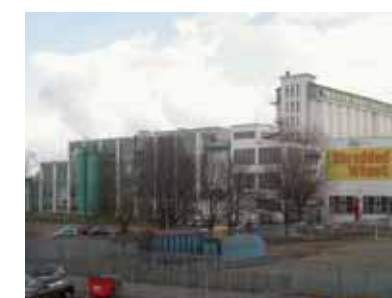
View of the 1920's buildings of Shredded Wheat factory
