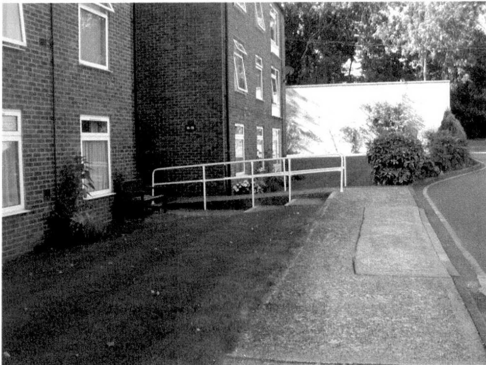
Front view looking at ramp and steps
