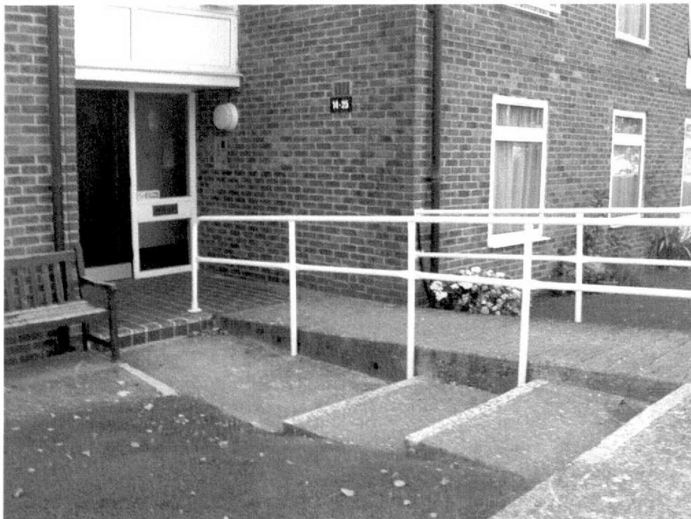
Front view looking at ramp and steps
