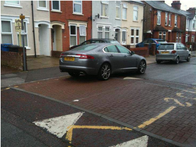
Raised table to provide new crossing for pedestrians near the train station:
