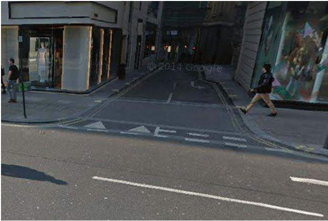
Raised table to improve pedestrian environment and discourage rat-running:
