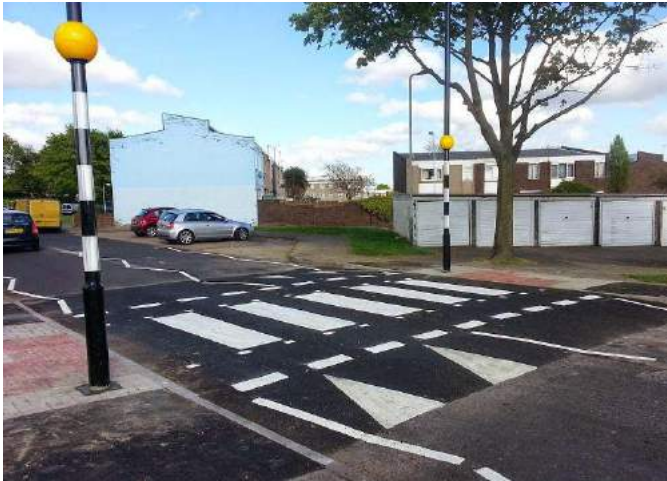
Raised Zebra Crossing to provide new pedestrian crossing near the post office:
