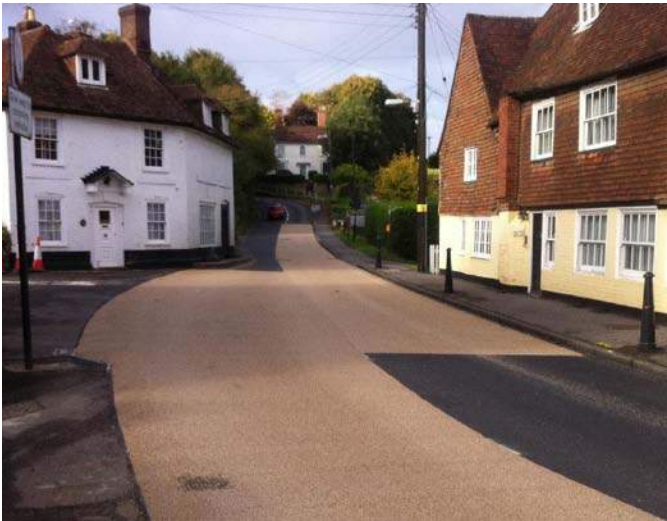
Buff Asphalt Surfacing at Plough Hill/Northaw Road/Station Road junction:
