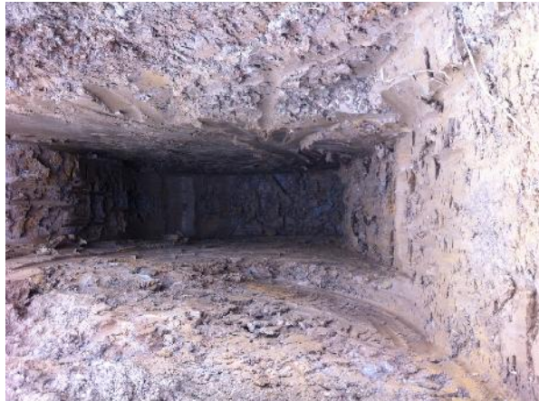
Photo 13: Excavation of trial pit TP03.
