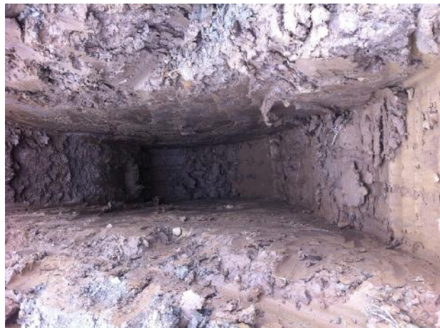
Photo 19: Excavation of trial pit TP06.
