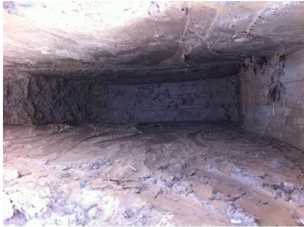
Photo 17: Excavation of trial pit TP05.
