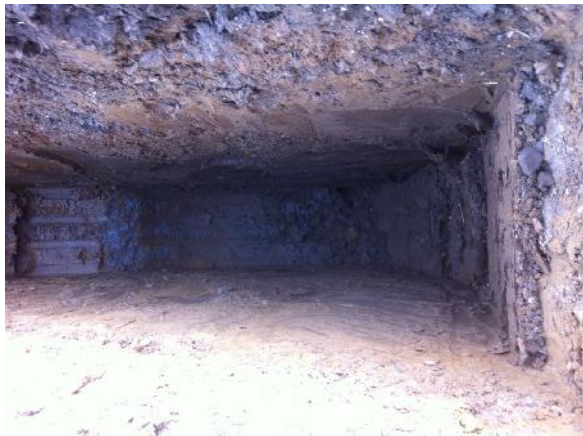
Photo 11: Excavation of trial pit TP02.
