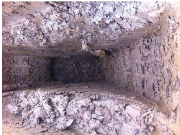
Photo 15: Excavation of trial pit TP04.
