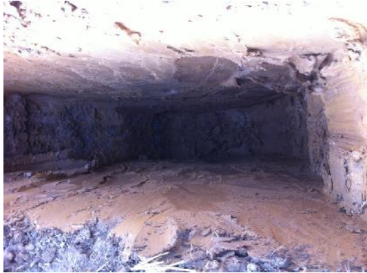
Photo 9: Excavation of trial pit TP01.
