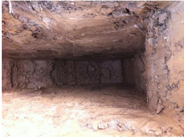
Photo 21: Excavation of trial pit TP07.
