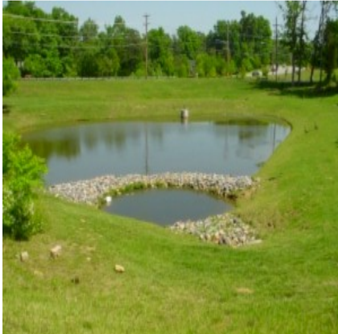
Figure 4d: Storage Basin
