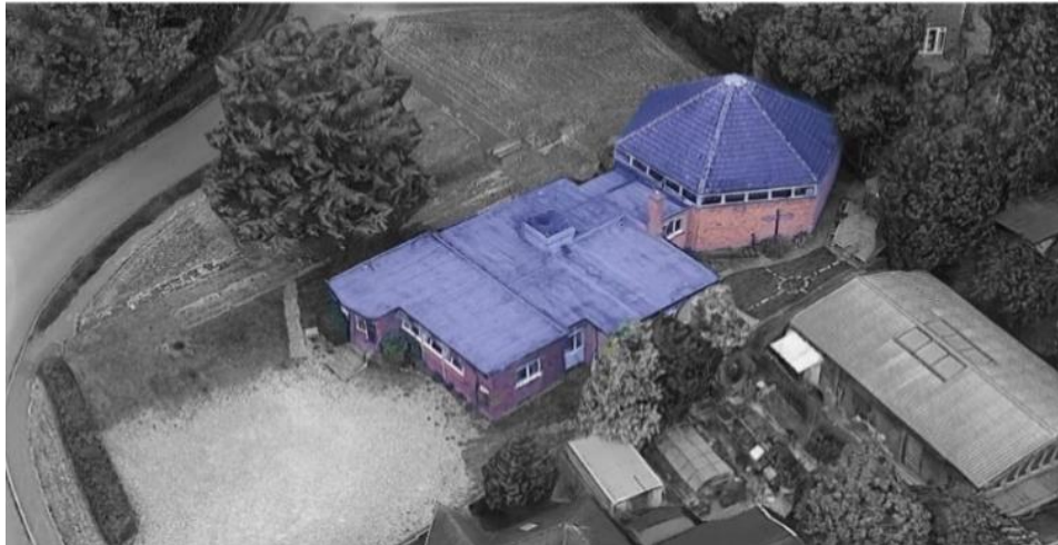
Figure 1: Aerial view of Warren Way, Digswell, Welwyn AL6 0DH (Copyright – Google Earth)
