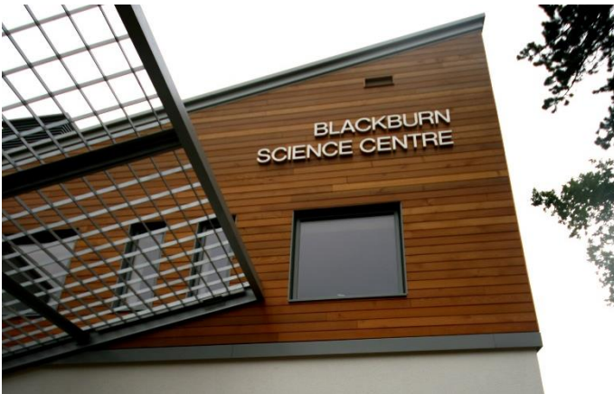
Walls: Coated Timber Boarding
