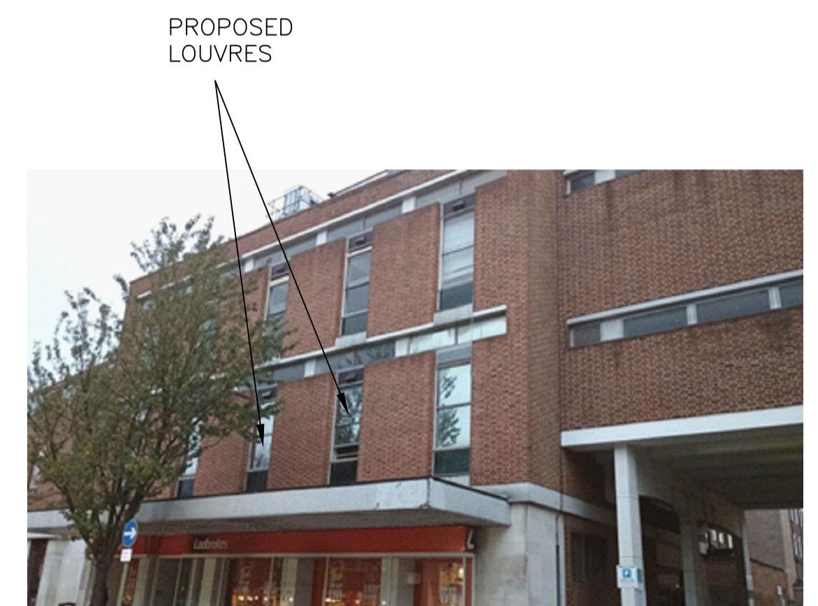
PHOTO OF EAST ELEVATION
