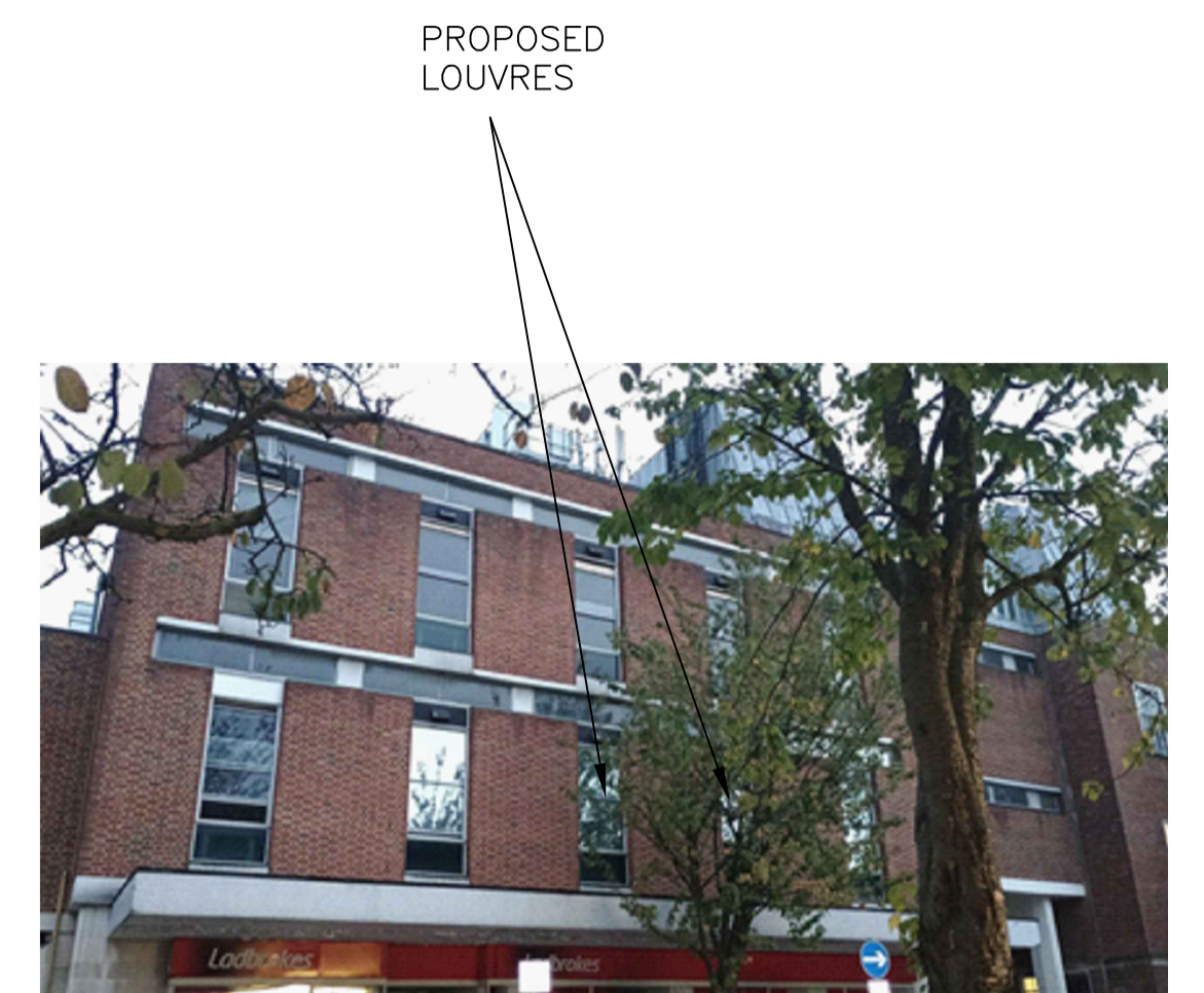
PHOTO OF EAST ELEVATION
