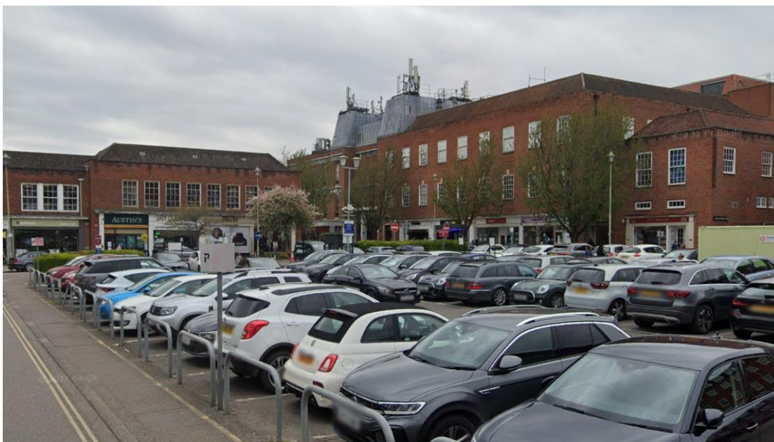
Northeastern elevation of site from Wigmores North.
