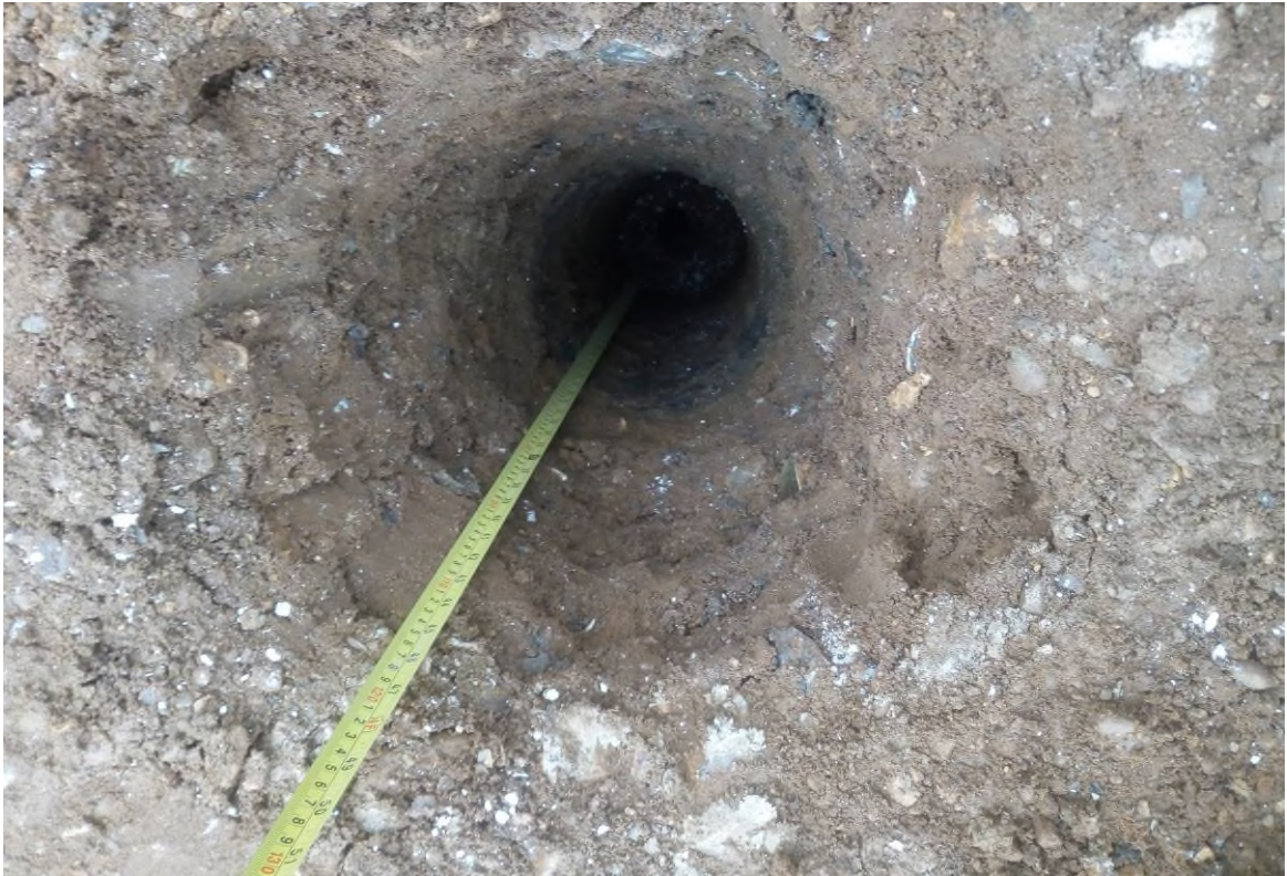
Hand dug pit (0.0-1.2mbgl) for BH03.
