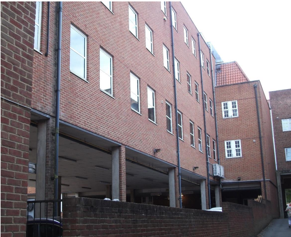
North Elevation taken from pedestrian passageway between Parkway and Wigmores North
