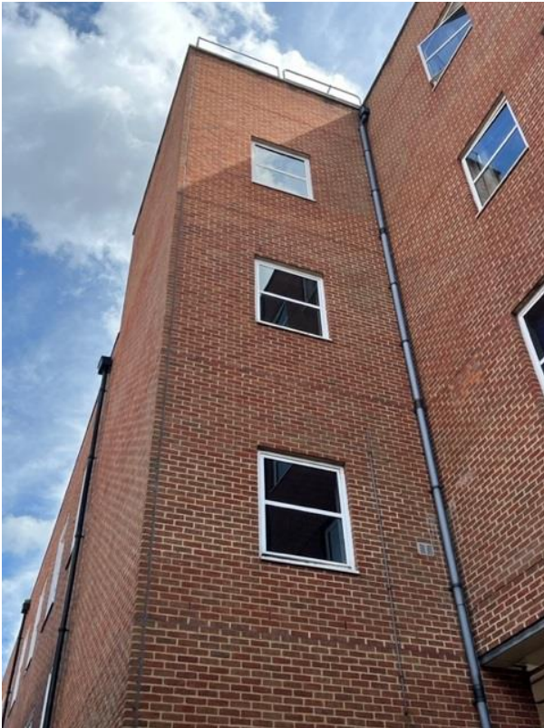
West Elevation taken from pedestrian passageway between Parkway and Wigmores North
