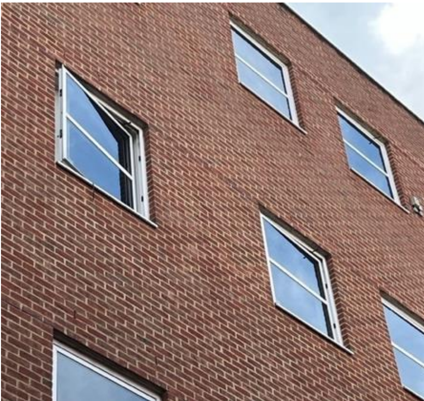
Close up of existing windows to be replaced.
