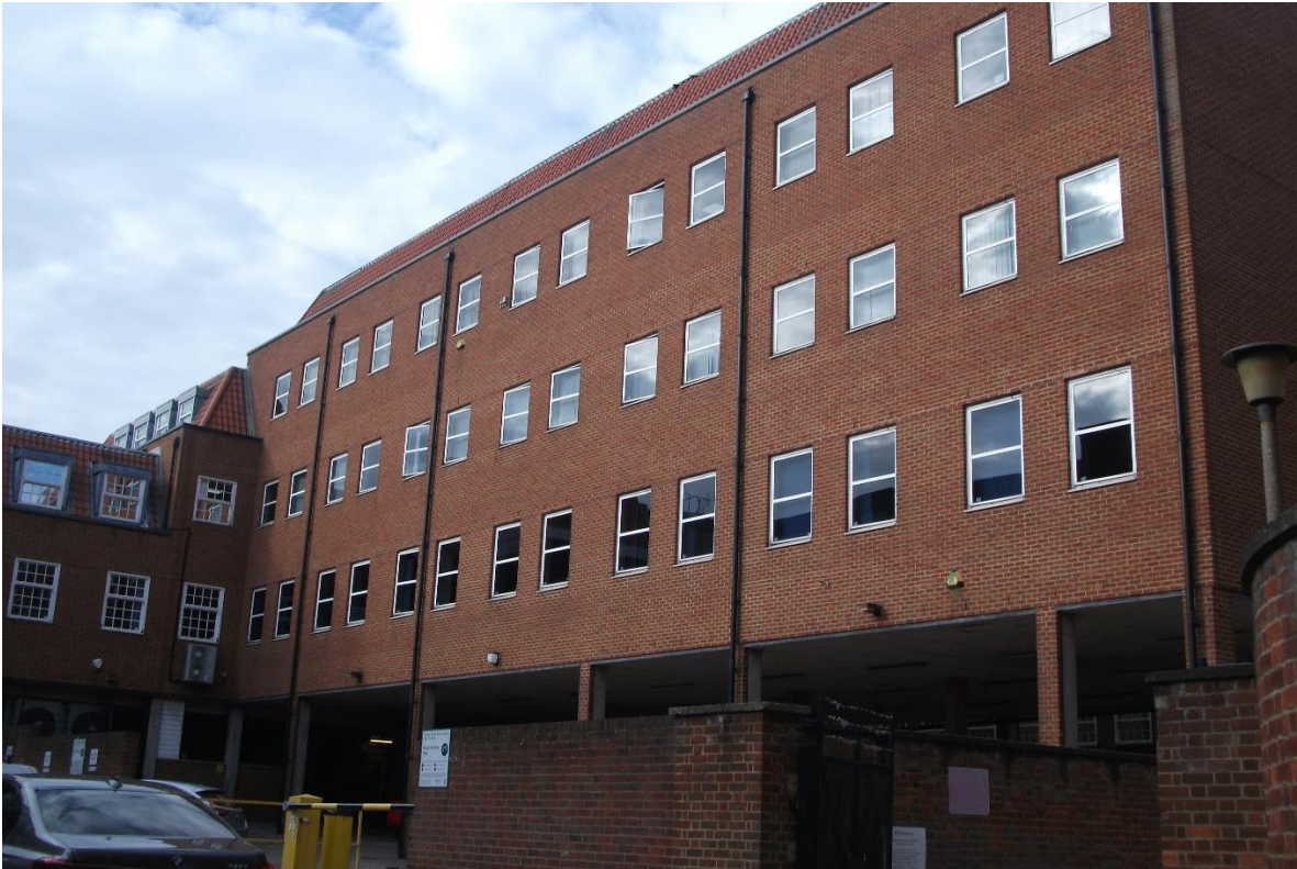
South Elevation taken from rear Carparking area accessed from Wigmores North
