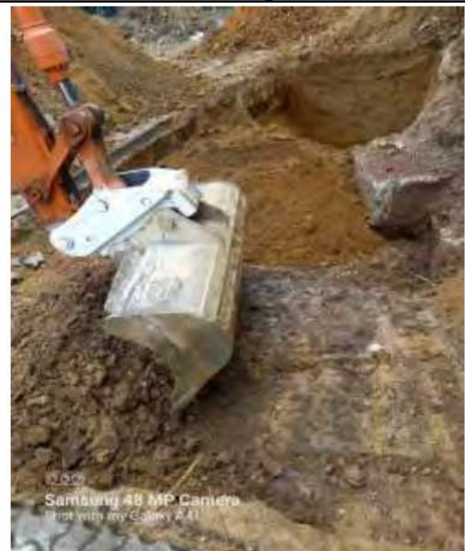
Plate 10. Ballast removed to dirty hardcore in the west
