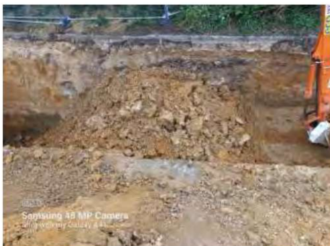
Plate 11. Clean subsoils placed in central hotspot excav.
