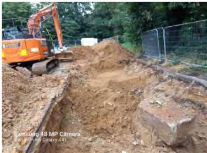
Plate 1. Ballast removal in the east
