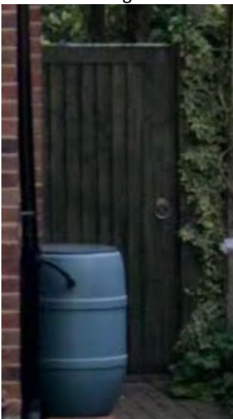
existing gate at no3
