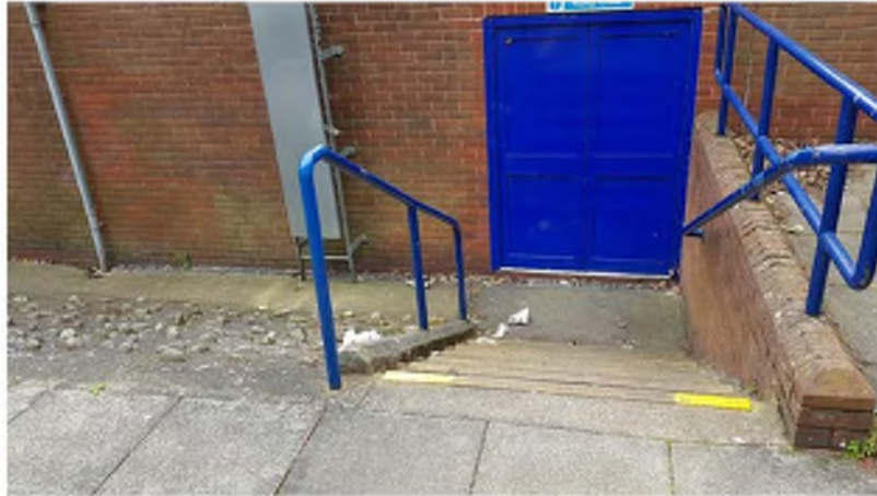
View of rear low level Fire Exit with Rear Lower Level Aco connecting into Gully2, which has allowed water to flood inside Roller City during very heavy rain
