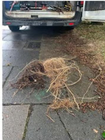
View of examples of debris / roots removed from SW drainage system
