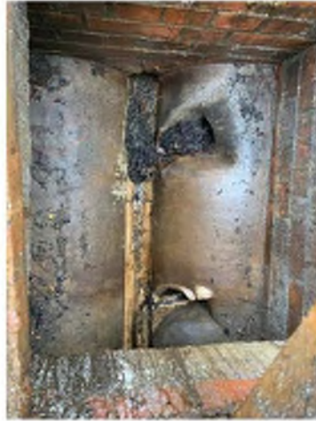
View of examples of debris / roots removed from SW drainage system
