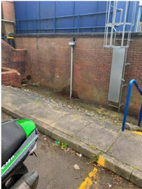
View of rear low level Fire Exit with Rear Lower Level Aco connecting into Gully2, which has allowed water to flood inside Roller City during very heavy rain
