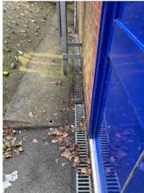
View of rear low level Fire Exit with Rear Lower Level Aco connecting into Gully2, which has allowed water to flood inside Roller City during very heavy rain
