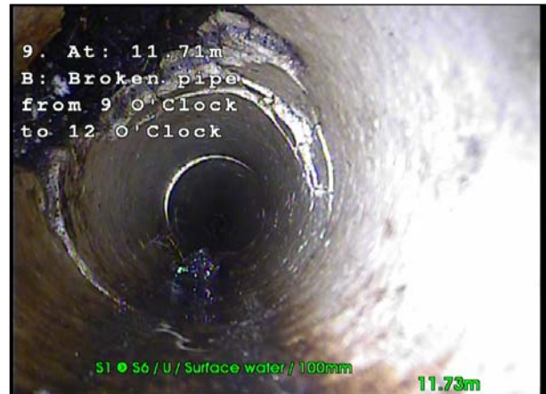
Photo: 23_23_191_A.jpg, 00:01:08 11.71m, Broken pipe, from 12 to 12 o'clock
