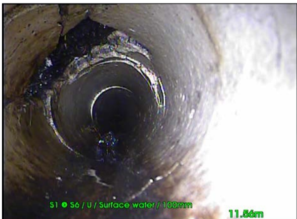
Photo: 23_23_486_A.jpg, 00:01:09 11.75m, Hole in drain/sewer, from 9 to 12 o'clock
