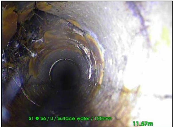
Photo: 22_22_488_A.jpg, 00:01:13 11.67m, Broken pipe, from 12 to 12 o'clock
