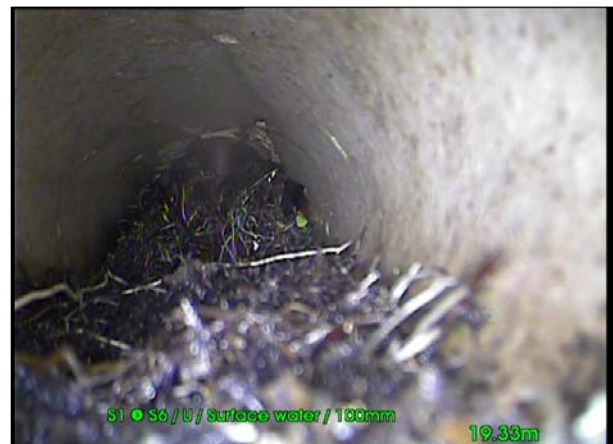
Photo: 22_22_179_A.jpg, 00:02:43 19.61m, Roots, mass 70 % cross-sectional area loss
