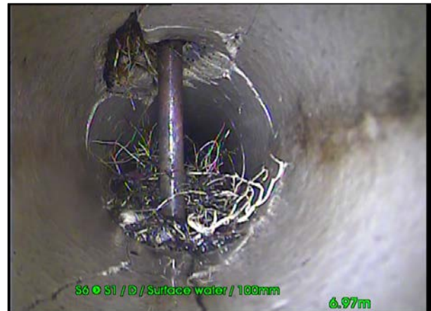
Photo: 25_25_585_A.jpg, 00:01:13 6.95m, Broken pipe, from 12 to 12 o'clock
