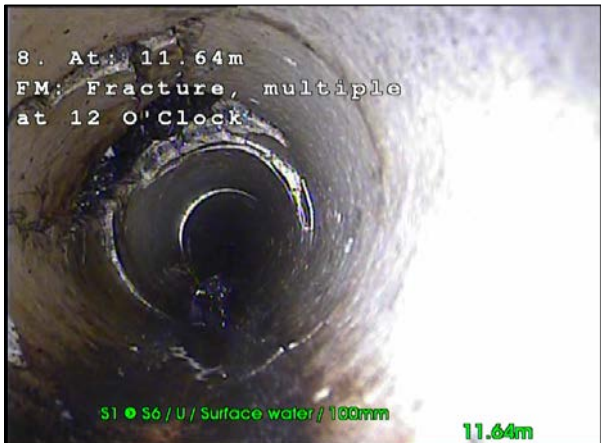
Photo: 23_23_190_A.jpg, 00:01:04 11.64m, Fracture, multiple, from 12 to 12 o'clock
