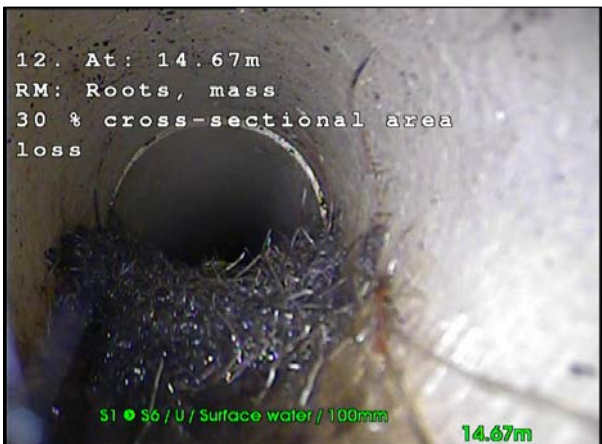
Photo: 22_22_176_A.jpg, 00:01:52 14.67m, Roots, mass 30 % cross-sectional area loss
