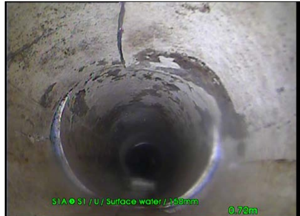
Photo: 30_30_499_A.jpg, 00:00:36 0.6m, Deformed sewer/drain, 5%
