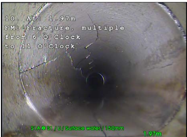
Photo: 30_30_257_A.jpg, 00:00:47 1.9m, Fracture, multiple, from 6 to 11 o'clock, Start
