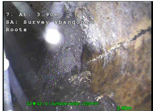
Photo: 32_32_274_A.jpg, 00:00:36 3.9m, Hole in drain/sewer, at 2 o'clock
