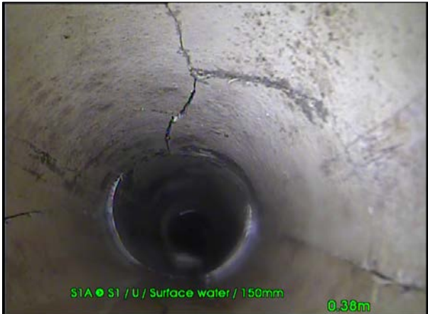
Photo: 30_30_498_A.jpg, 00:00:30 0.3m, Fracture, multiple, from 12 to 12 o'clock
