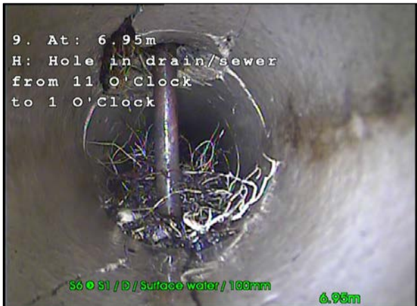
Photo: 25_25_212_A.jpg, 00:01:12 6.95m, Hole in drain/sewer from 11 O'Clock to 1 O'Clock
