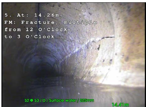
Photo: 31_31_264_A.jpg, 00:01:02 14.26m, Fracture, multiple from 12 O'Clock to 3 O'Clock
