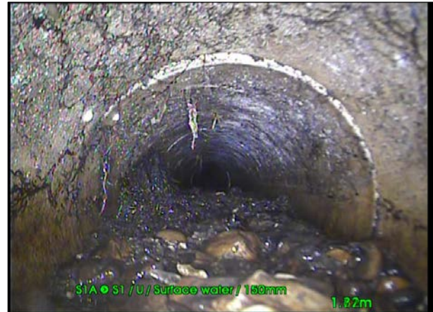
Photo: 28_28_241_A.jpg, 00:00:16 1.82m, Settled deposits, fine, 30% cross-sectional area loss, Start
