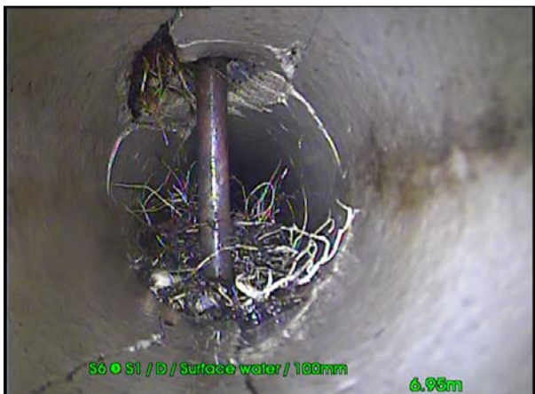
Photo: 25_25_213_A.jpg, 00:01:18 6.97m, Fracture, multiple at 12 O'Clock
