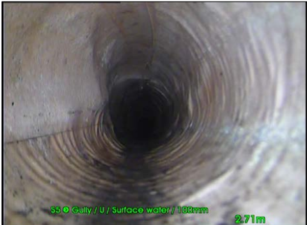
Photo: 2_2_4_A.jpg, 00:00:31 2.79m, Deformed sewer/drain, 10%
