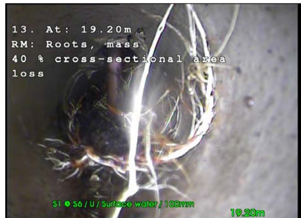
Photo: 23_23_195_A.jpg, 00:02:06 19.2m, Roots, mass 40 % cross-sectional area loss
