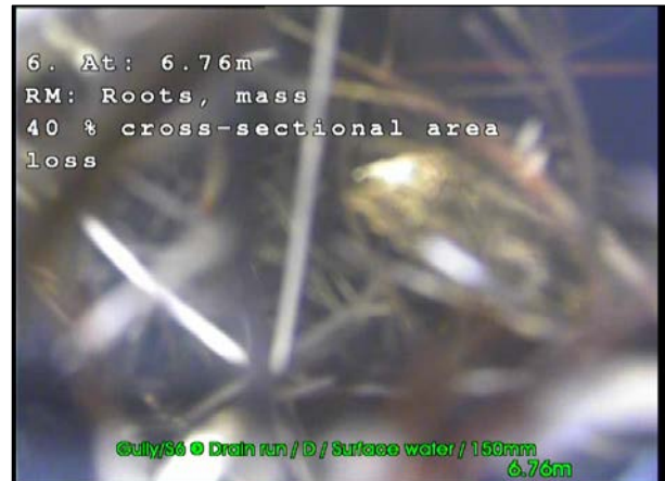
Photo: 17_17_114_A.jpg, 00:01:36 6.76m, Roots, mass 40 % cross-sectional area loss
