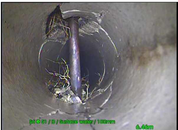
Photo: 27_27_586_A.jpg, 00:00:59 6.46m, Hole in drain/sewer, from 11 to 1 o'clock
