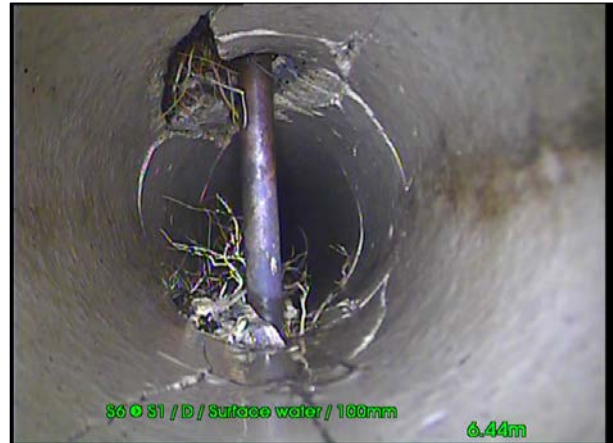
Photo: 27_27_236_A.jpg, 00:01:03 6.46m, Other obstacles protruding through wall, from 12 to 6 o'clock, 95% cross-sectional area loss
