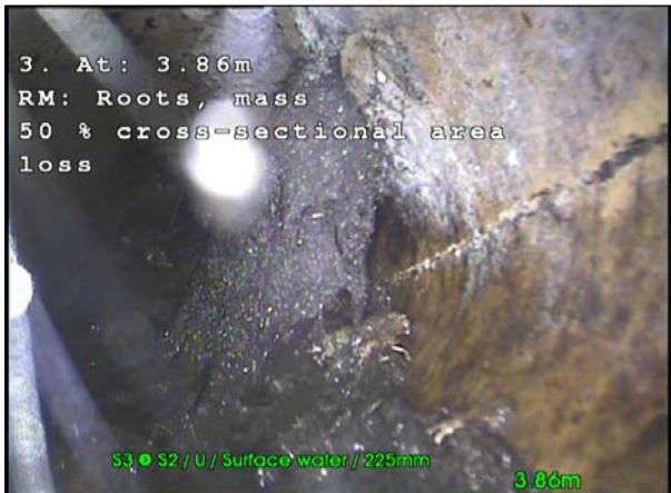
Photo: 32_32_272_A.jpg, 00:00:20 3.86m, Roots, mass 50 % cross-sectional area loss
