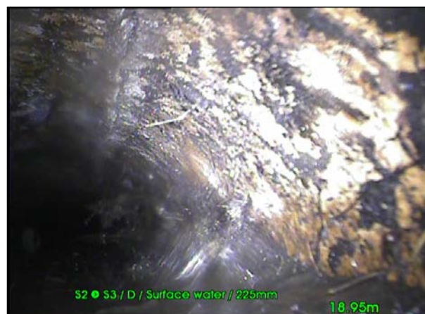
Photo: 31_31_506_A.jpg, 00:02:11 18.82m, Roots, mass, 50% cross-sectional area loss
