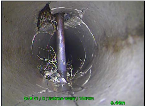
Photo: 27_27_232_A.jpg, 00:00:56 6.46m, Broken pipe, from 12 to 12 o'clock
