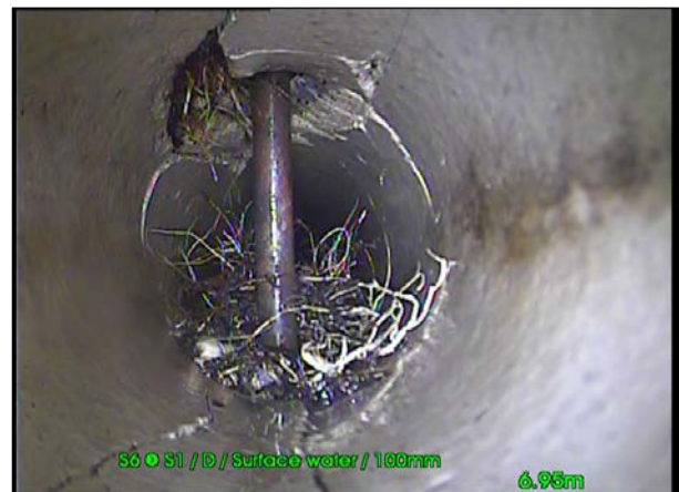
Photo: 25_25_214_A.jpg, 00:01:19 6.97m, Other obstacles protruding through wall, from 12 to 6 o'clock, 95% cross-sectional area loss (rod / spike)
