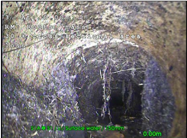
Photo: 28_28_240_A.jpg, 00:00:03 0m, Roots, mass 30 % cross-sectional area loss
