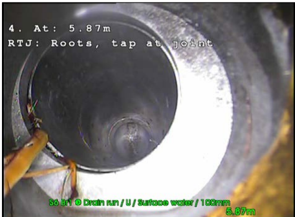
Photo: 11_11_67_A.jpg, 00:00:56 5.87m, Roots, tap at joint
