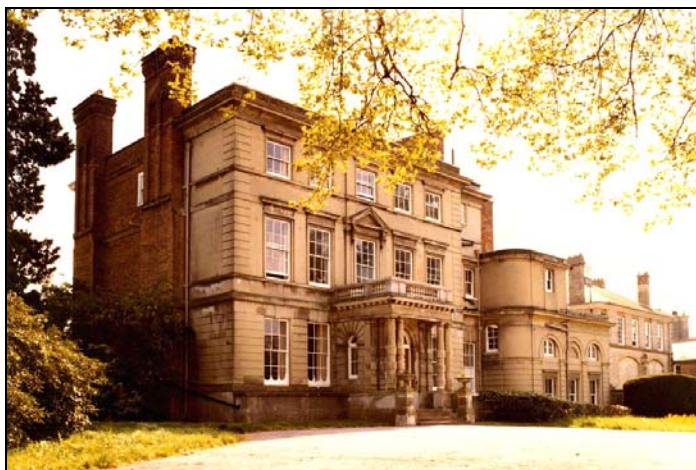
Northaw Place viewed from the northeast (1981)
