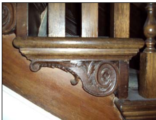
Detail of stair tread bracket
