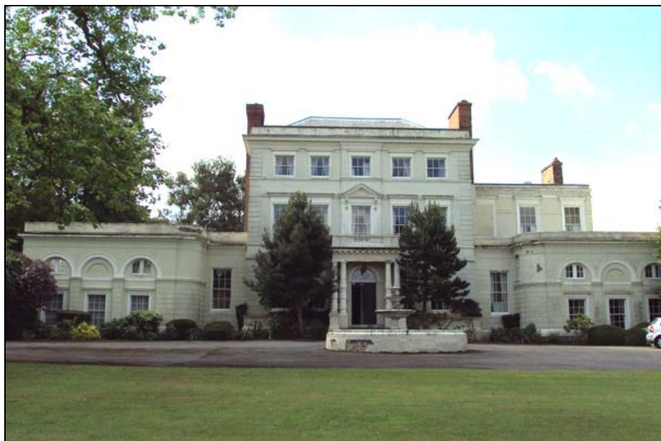
Northaw Place; front (north) elevation
