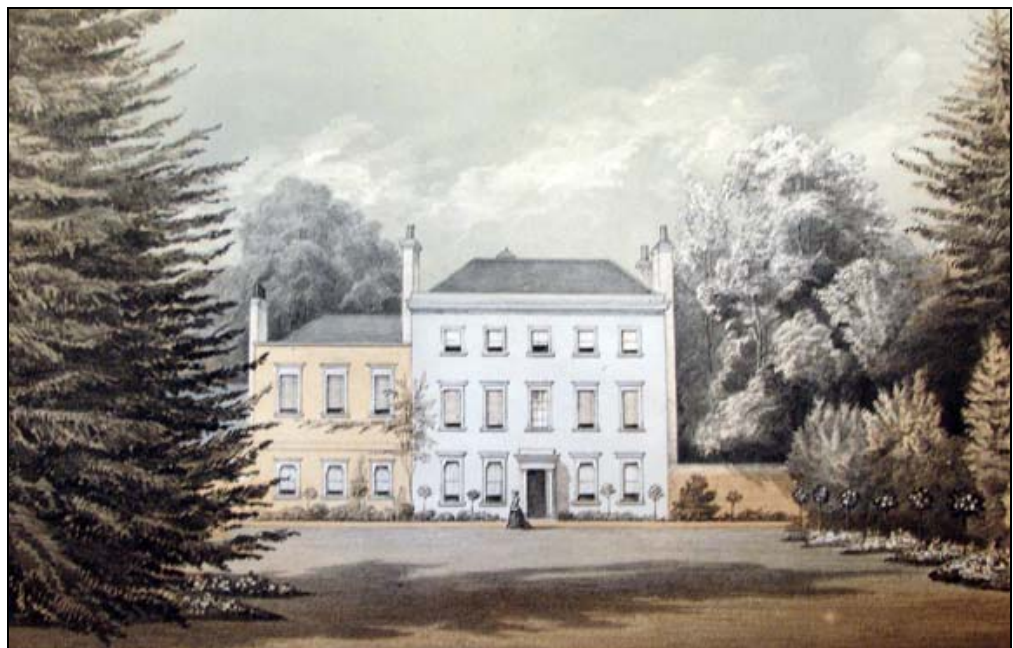
Figure 7. Northaw Place, rear elevation in c. 1867 (HALS)
