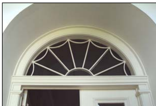
19 th century fanlight above front door
